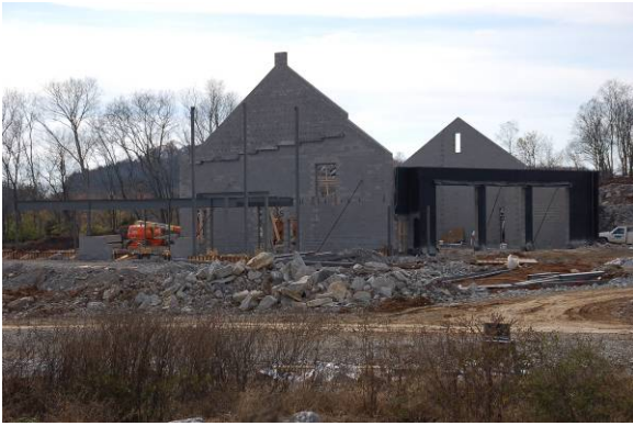
Station #6 construction in November 2006
