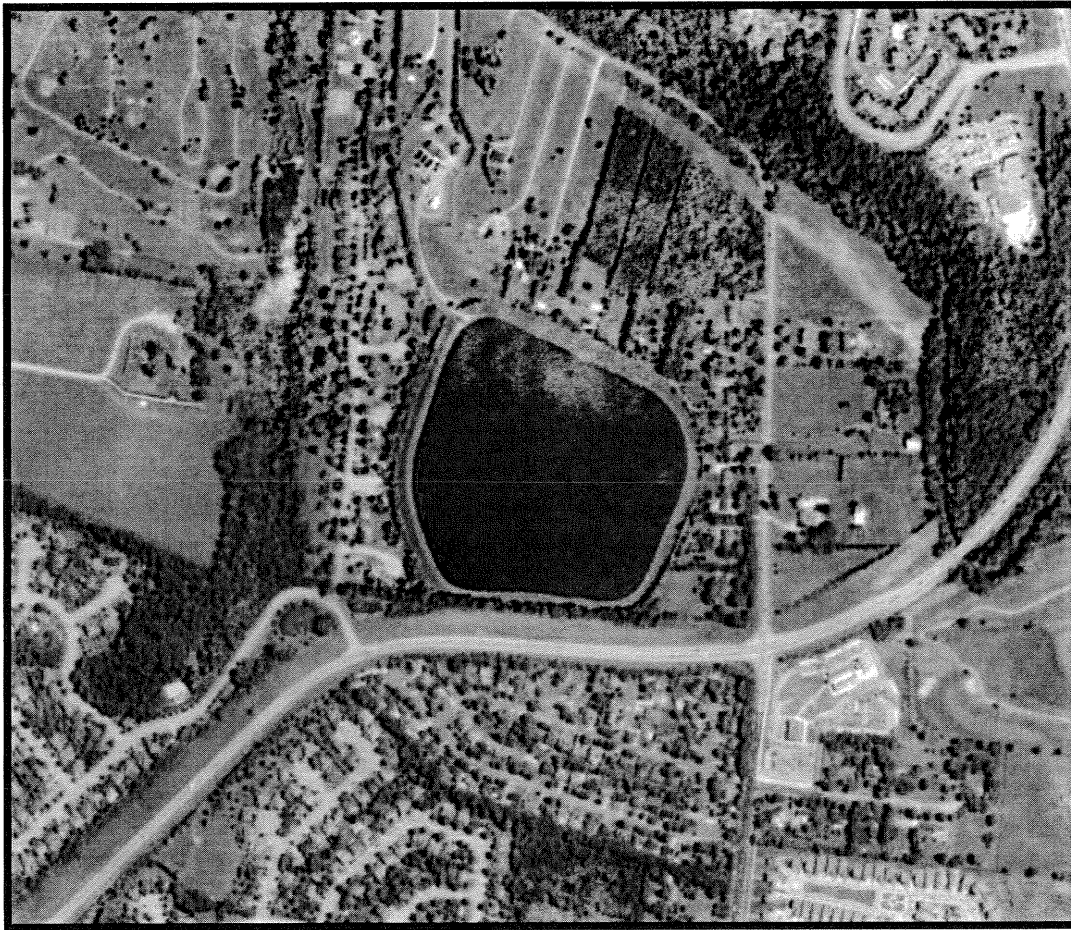
Photo of Franklin Raw Water Reservoir provided by Google Earth
