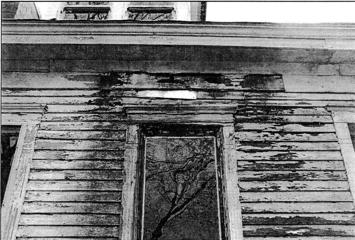
Most of the outside and inside damage was caused from the gutter system leakage over years
