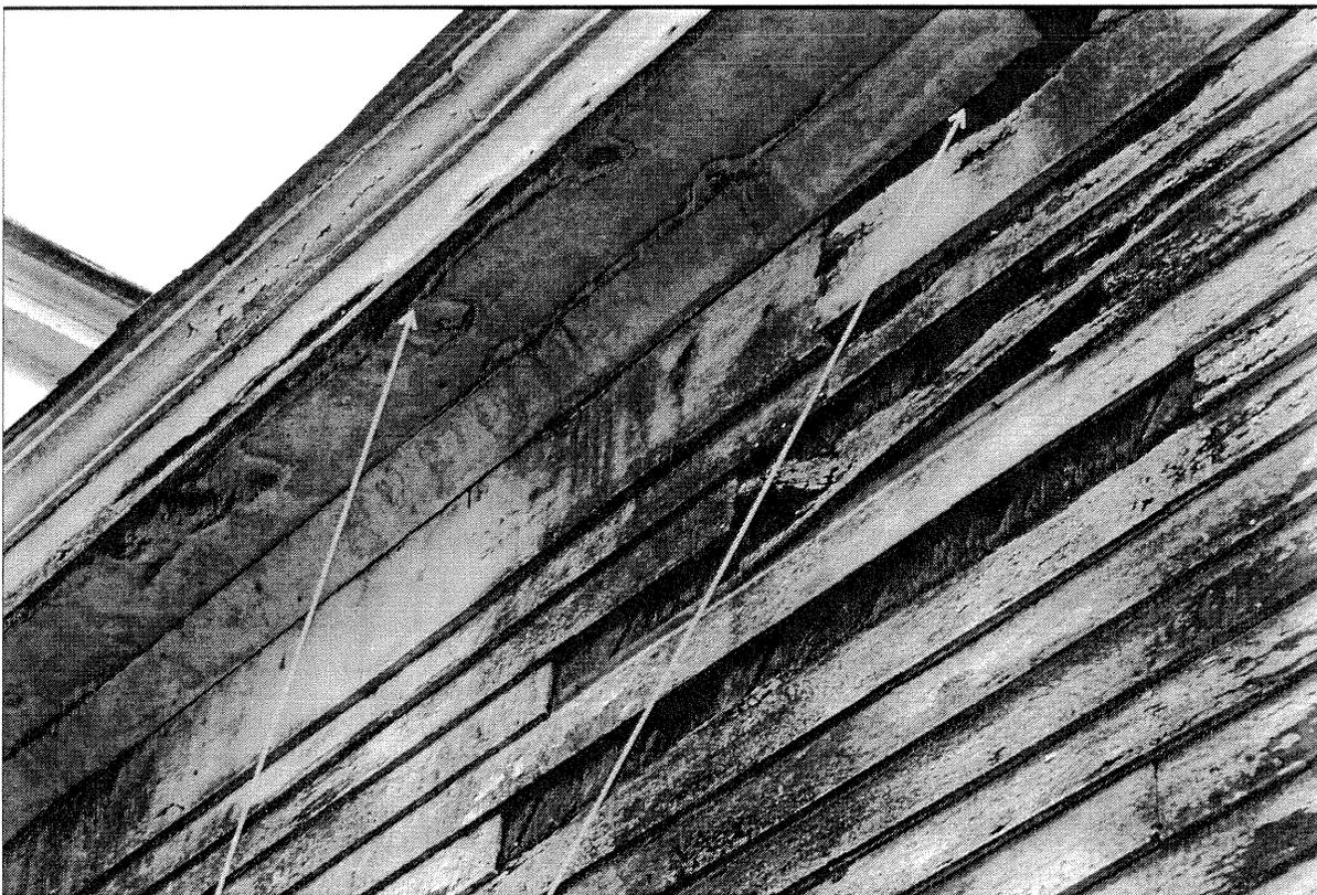
Box gutter system has failed letting water go down the middle of wall
