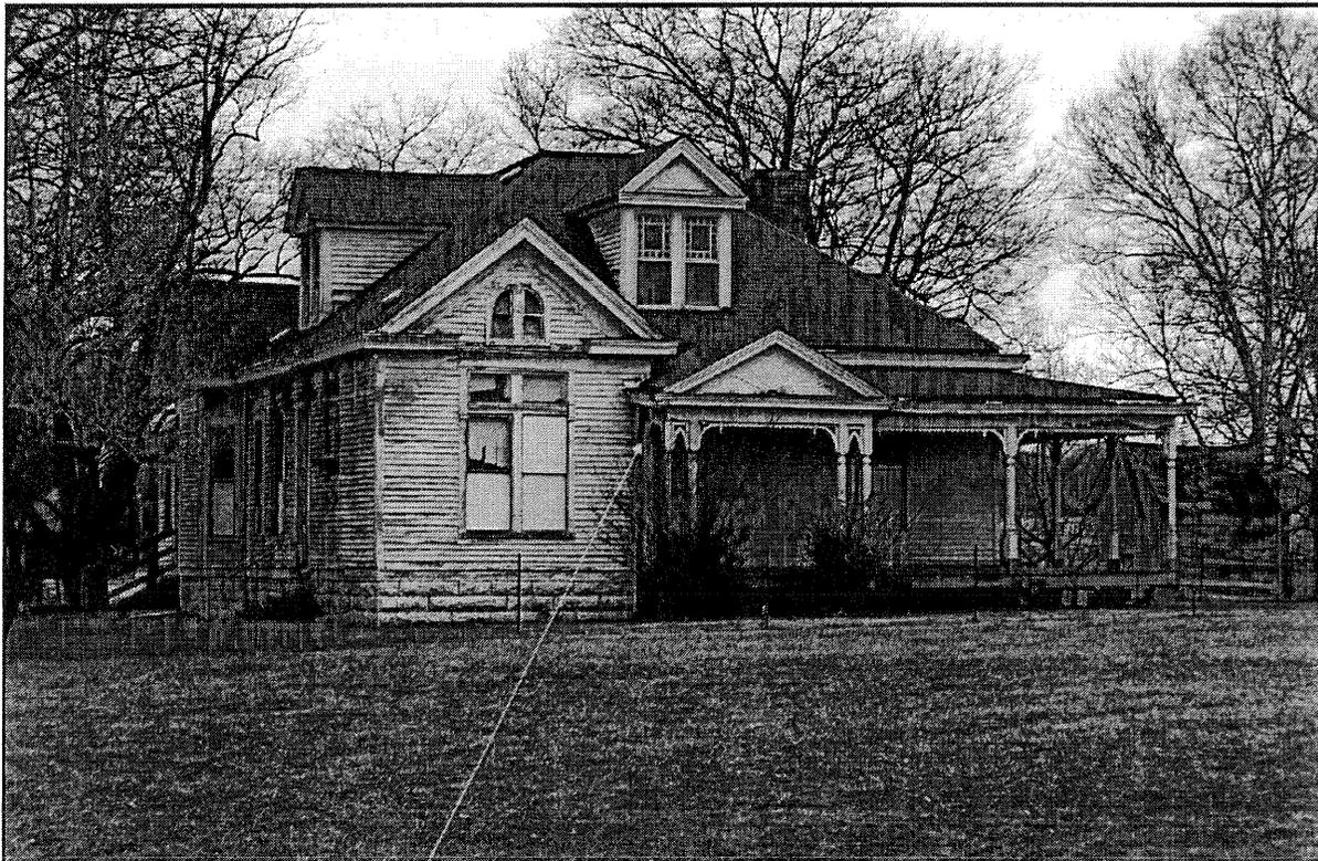
Front porch has settled and a lot of the trim has separated. This has allowed weather to cause dry rot of gutter boards, framing and soffits. This separation from settling has happened all the way around the home.
