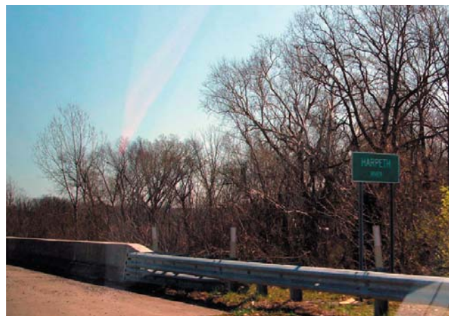
Photo 3.24 Existing Harpeth River Crossing
