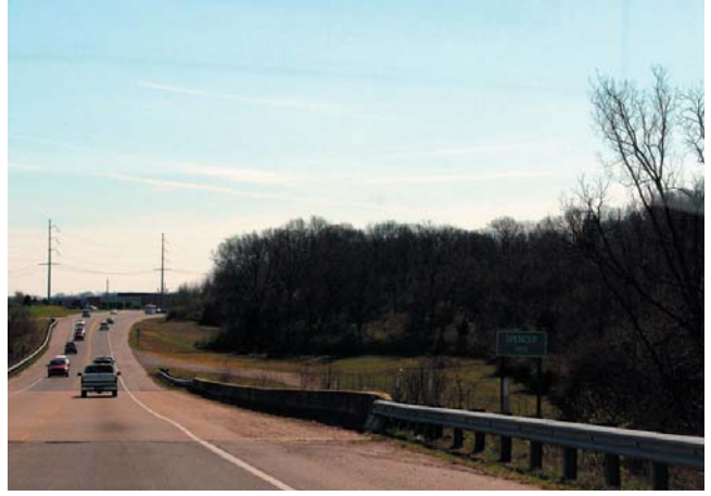
Photo 3.2 Approaching Cool Springs Blvd., Roper's Knob
