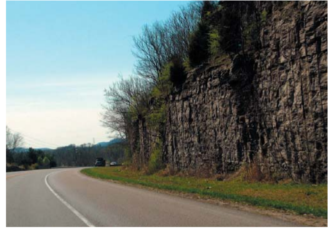
Photo 3.4 Typical rock cut
