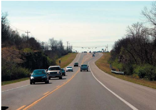
Photo 3.3 Approaching Highway 96/Murfreesboro Road
