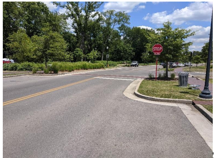
intersections and create shorter crossing distances for pedestrians. The reduction in lane width encourages motorists to slow down when driving through the intersection. (3 rd Ave / 4 th Ave, Franklin TN)
