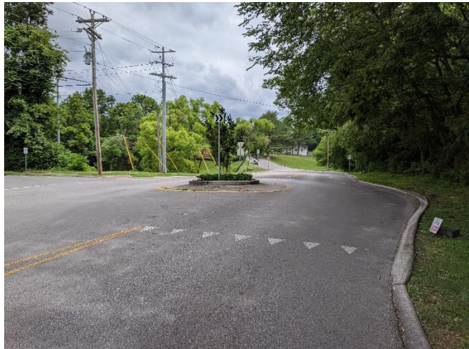
A traffic circle creates a horizontal deflection in the roadway, which causes motorists to slow down as they travel through the intersection. (Twin Oaks Drive / Birchwood Circle, Franklin TN)
