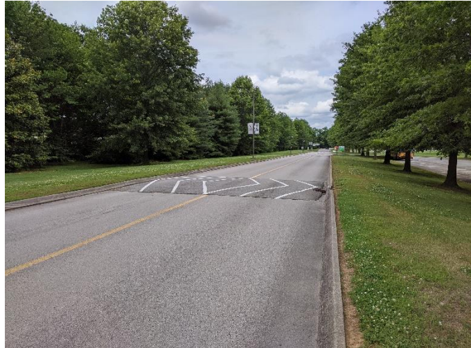
The speed table/hump that may be used in the City of Franklin is 22 feet long and three inches high. (Vera Valley Drive, Franklin TN)
