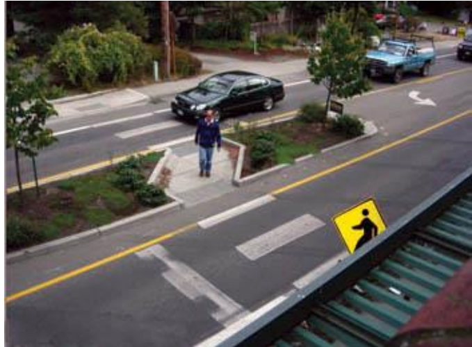
Raised medians reduce the width of the adjacent travel lanes. (Source: Google)
