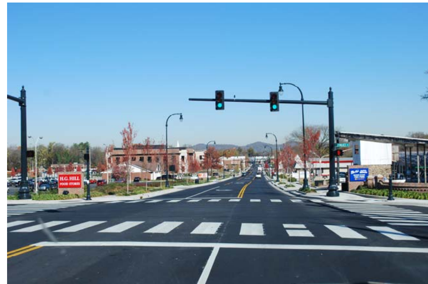
Columbia Avenue AFTER Streetscape.
