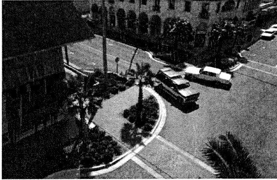
Curb extensions reduce the width of the roadway at intersections and create shorter crossing distances for pedestrians. The reduction in lane width encourages motorists to slow down when driving through the intersection.
