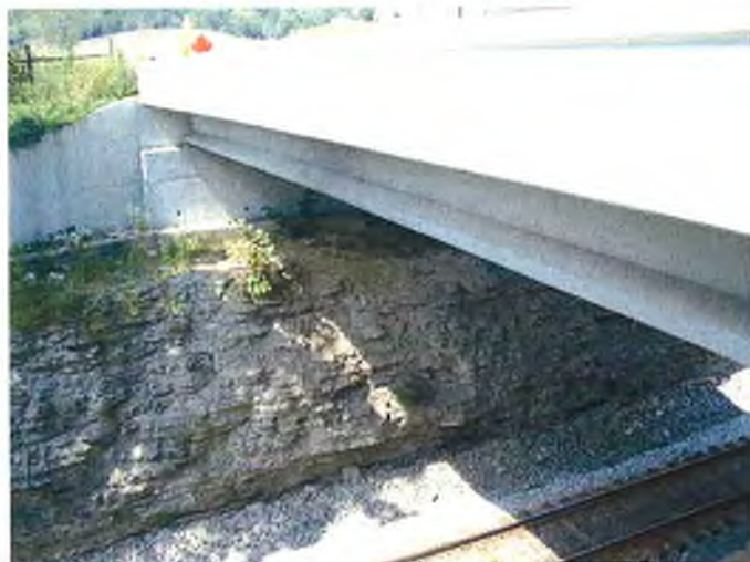
Photo 1 - Existing McEwen Road, 2-lane Bridge
