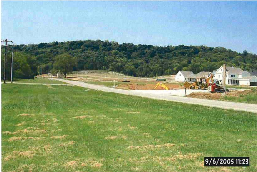
7) View west along existing McEwen Road near Station 505+00
