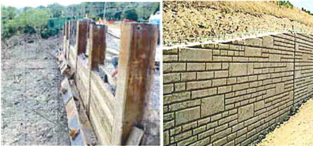
Photo 3 - Raw & Faced Soldier Pile Wall
