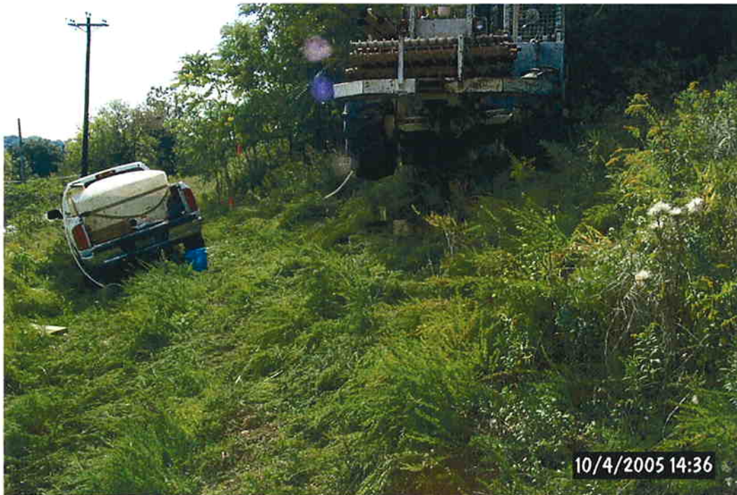
6) Coring setup on side slope near STA 473+00
