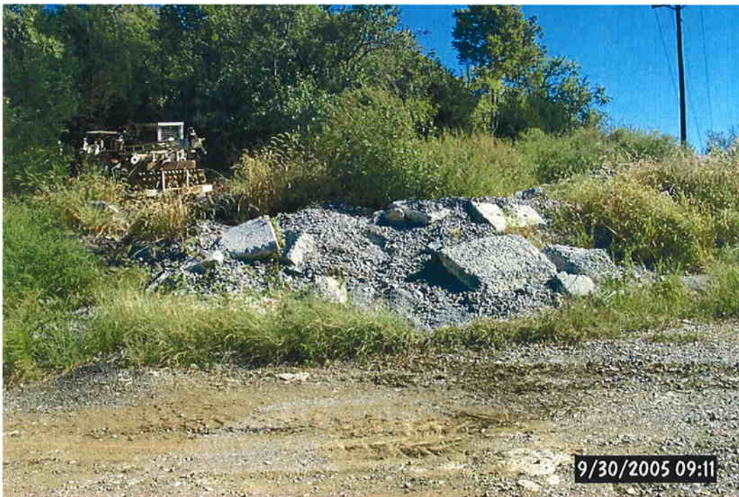
4) Debris near STA 468+00
