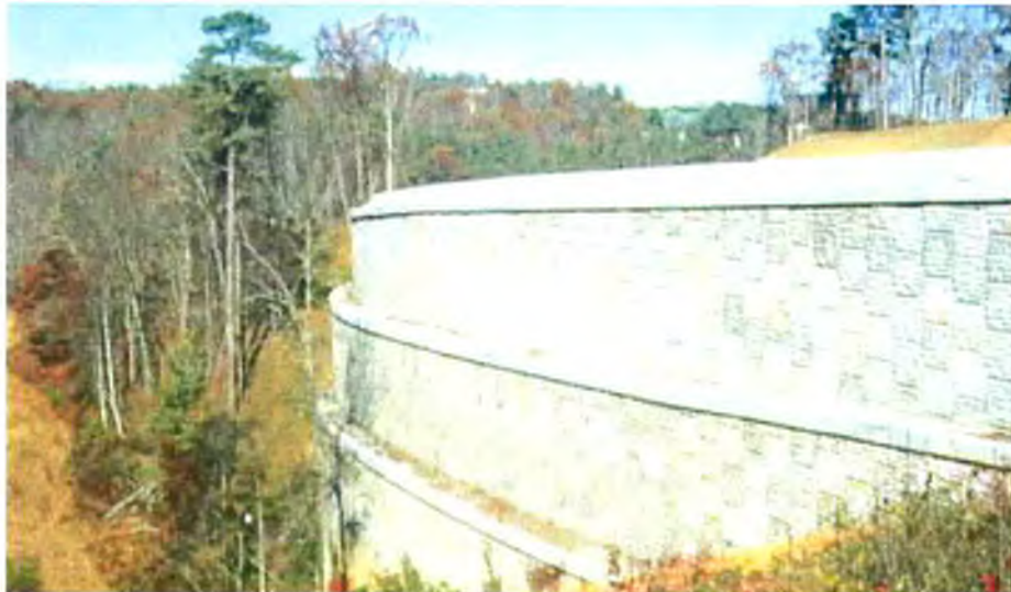
Photo 2 - Ashlar Stone Reinforced Earth Wall
