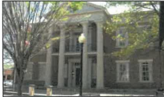
Court House - used as a post-battle hospital.
