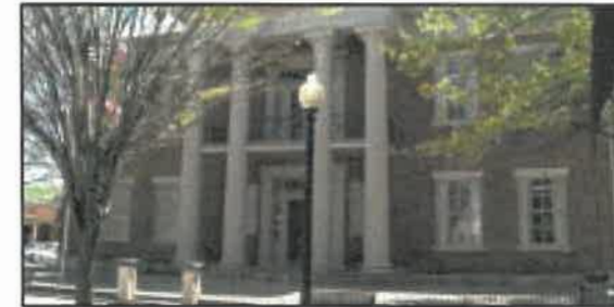
The fact that the historic County Courthouse served as a hospital after the Battle of Franklin adds to its appeal as a visitors center. Its location would also leverage economic benefits to downtown.
