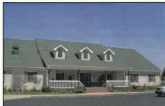
The Club House's design eludes to the vernacular rural architecture of 19th-century Franklin.
