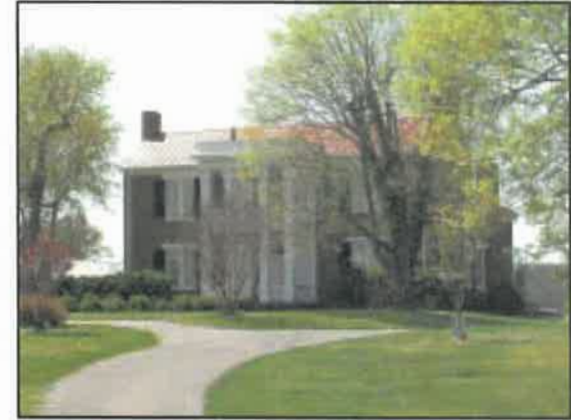
Because the Harrison House is privately owned and not open to the public, a visual connection should be afforded from the top of Winstead Hill.
