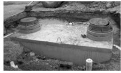
**Grease Trap**- make sure flow restrictor installed and properly vented.
