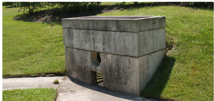
Figure 2: A typical outlet structure
