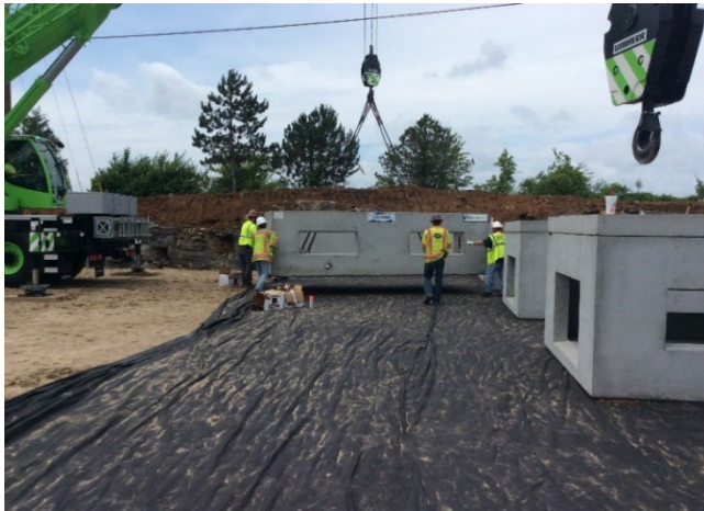
Figure 9: Installation of a concrete vault underground detention system.
