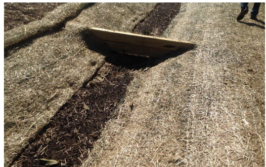
Figure 7: Wooden check dam in a water quality swale
