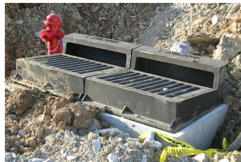
Vane grate for curb and gutter section
