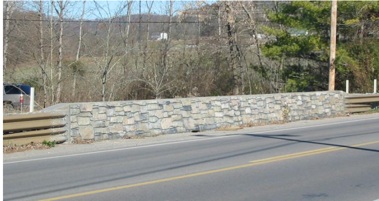
Bridge Rail Barrier
