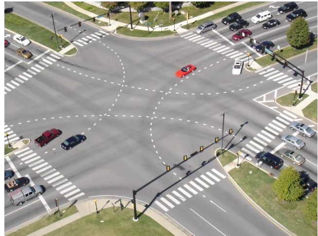
Channelization at intersection
