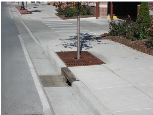
Vertical combined curb and gutter
