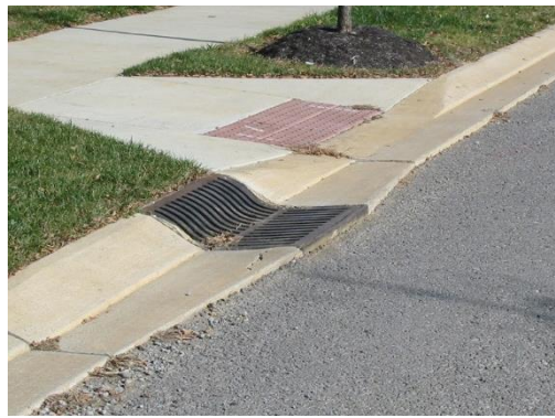
Rollover curb with grate transition
