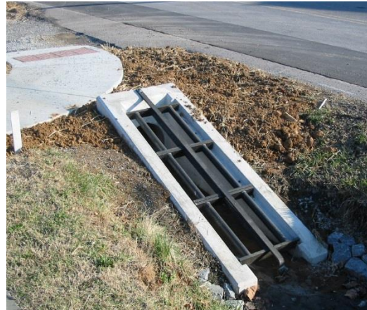
TDOT Safety Endwall
