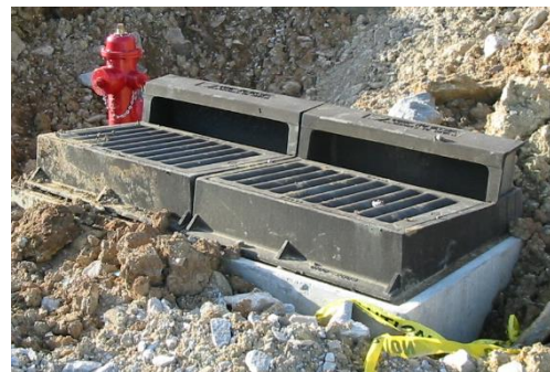
Vane grate for curb and gutter section
