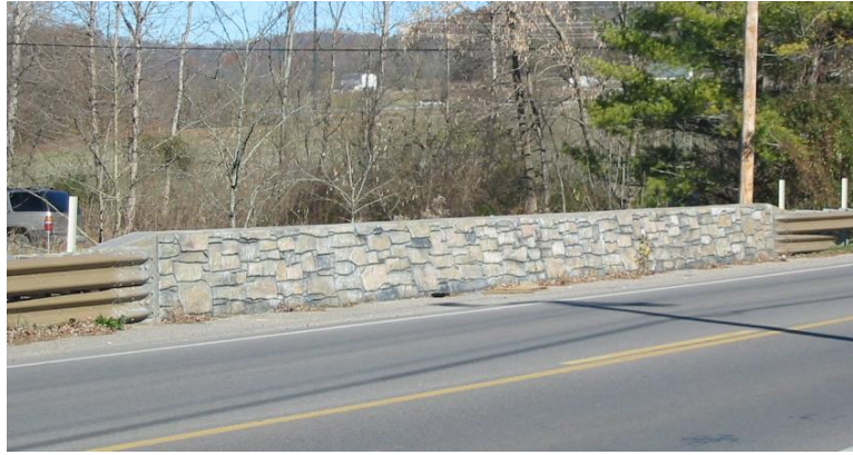
Bridge Rail Barrier
