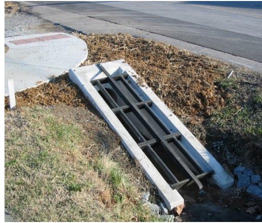
TDOT Safety Endwall
