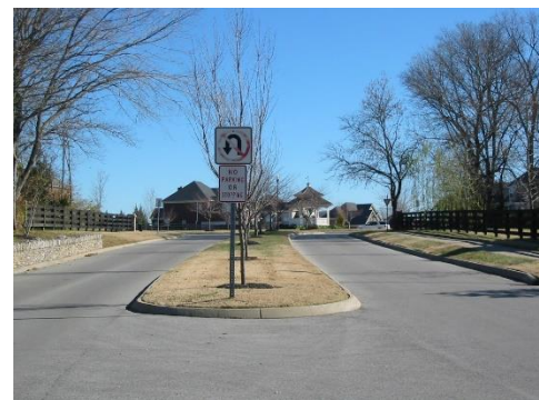
Typical Raised Median
