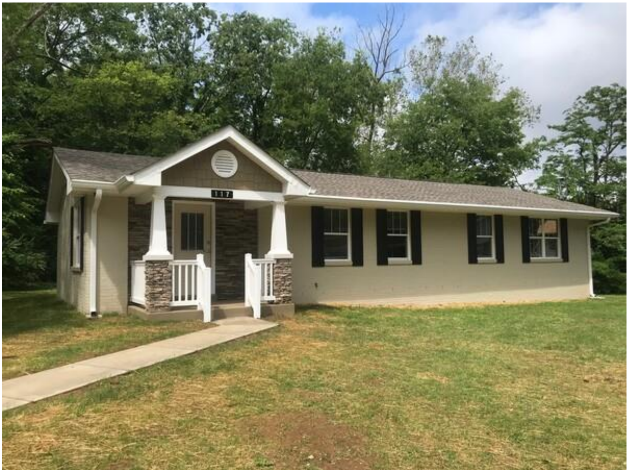
Spring Street Johnson Circle Renovation
