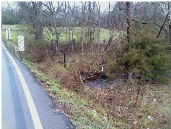
This was the site of the wreck on Cross Keys Rd. in rural Williamson County.
