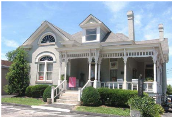
This house at 206 Main Street shows a mix of influences. Queen Anne features include its irregular plan and various surface planes, corbelled chimneys, and milled porch trim and posts.
