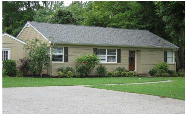
On Everbright Avenue, also, Ranch houses were popular later additions. This dwelling is at 109 Everbright Avenue.
