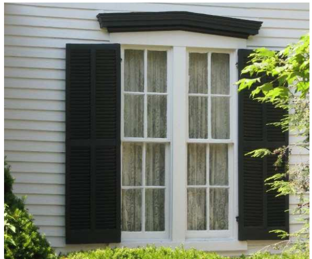
Clear glass panes were typical in historic windows, like these at 1010 West Main Street.
