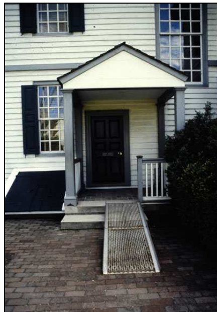
The use of temporary or portable ramps such as this one has minimal visual impact on a dwelling.
