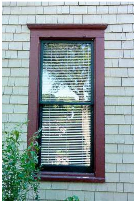
A old growth wood window (left) has a longer life expectancy than most new vinyl windows.
