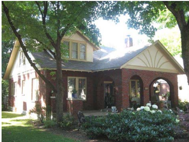
The projecting brick porch with arched openings at 916 Fair Street contributes to its Tudor Revival style and historic character.
