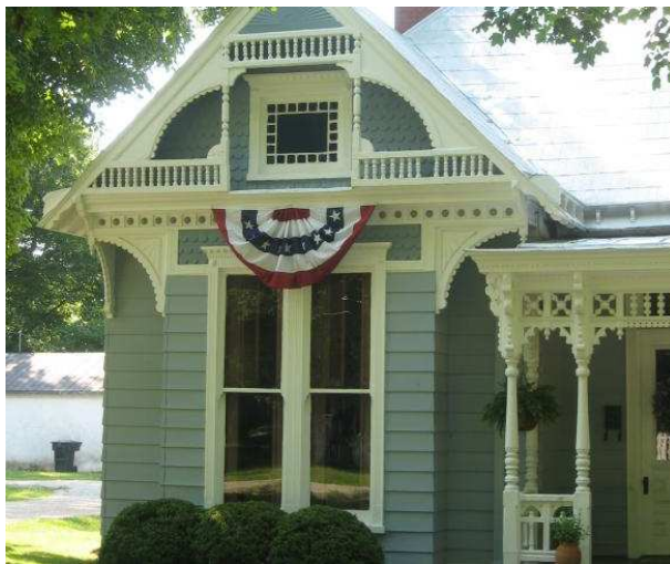
Fixed windows with decorative glass and one-over-one double-hung windows like these on 1002 Fair Street were popular during the Victorian era.
