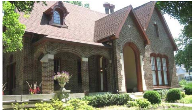
The contrast between various exposed masonry elements and painted wooden elements contributes to the Tudor Revival character of this house.
