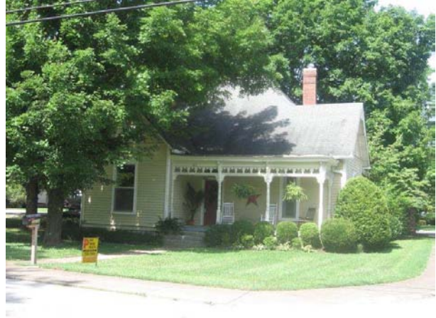
The appearance of the house and setting at 1312 Adams Street is typical of the district. The house has one story, limited detailing, frame construction, and a gabled and hipped roof. Its yard includes grass and trees, and adjoining the lot are the sidewalk and street.
