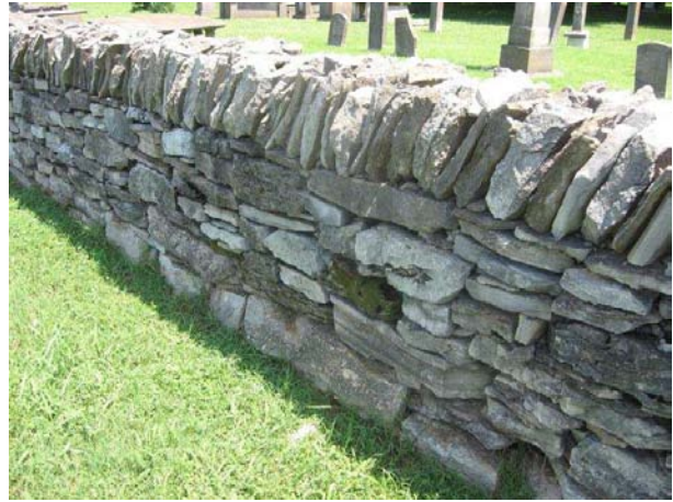
Stacked stone walls like this one at the City Cemetery are a key characteristic of the district cemeteries.
