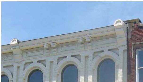
Metal cornices like the one on 334 Main Street were often used on commercial buildings from the late 1800s.
