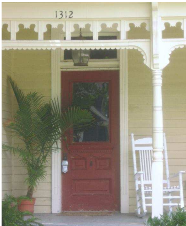
This historic door and transom at 1312 Adams Street are typical 19th- and early 20th-century entry elements.
