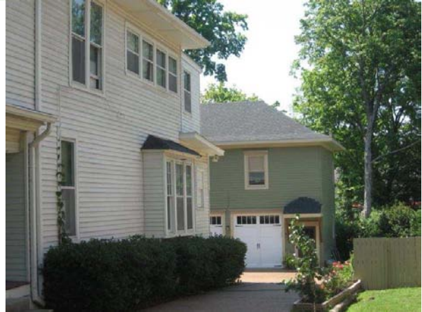
The garage apartment at 1016 West Main Street demonstrates traditional doors and other details.
