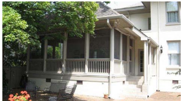
Shown at 238 Third Avenue South is a model for enclosing a porch with minimal alteration or obstruction to its structural or decorative elements.
