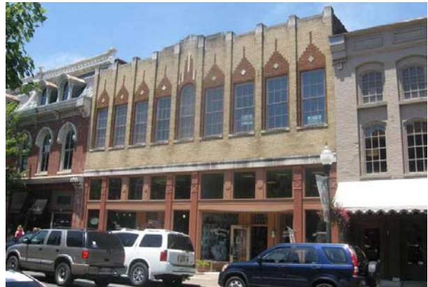
Adding additional architectural features to buildings like this one at 342-244 Main Street would detract from their original styles and appearance.
