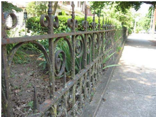
Metal fences like the one at 908 West Main Street were popular Victorian landscape elements.
