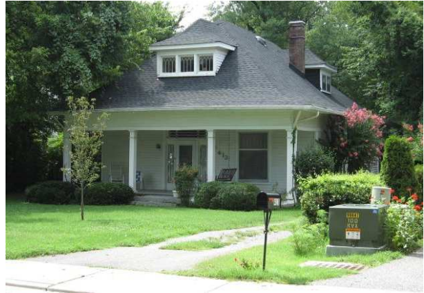
The house at 413 Boyd Mill Avenue is an example of the vernacular Pyramid Square plan.
