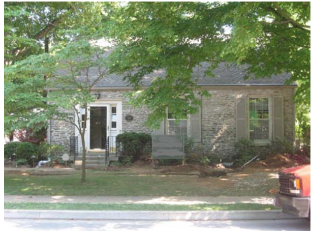
This property, at 921 Fair Street, reflects the Colonial Revival style in its symmetry and entrance with side-lights.
