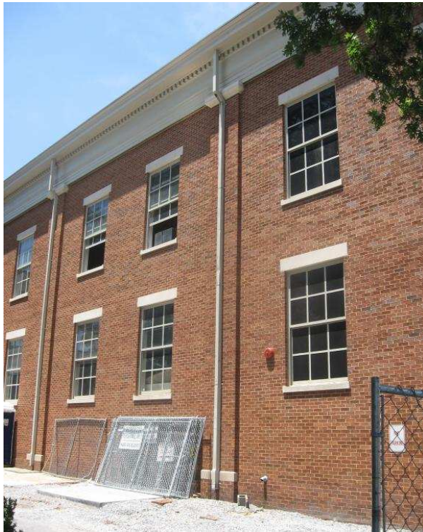
Gutters and downspouts, like these on the courthouse, help protect buildings from water damage.
