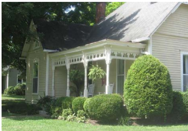
The Queen Anne-influenced porch trim at 1312 Adams Street is an important visual component of the house.
