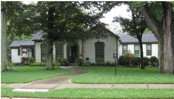
The arched openings and window hoods at 114 Lewisburg Avenue give this house an Italianate feel.
