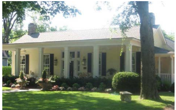
The number and placement of the windows at 1008 Fair Street helps create the house's symmetry.
