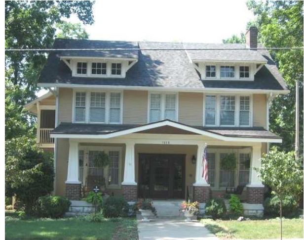
The central placement of this front entrance contributes to the symmetry that defines the house at 1018 West Main Street; removing or altering it or adding additional entrances would damage the house's character.
