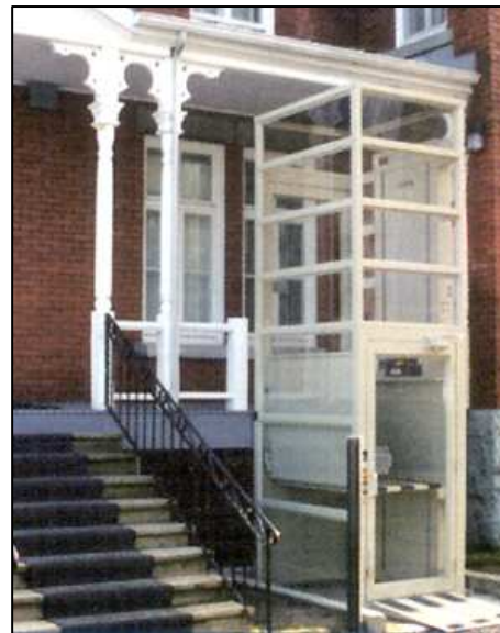
Wheelchair lifts may be appropriate to access rear elevations of commercial buildings or dwellings now used for commercial or office space.
