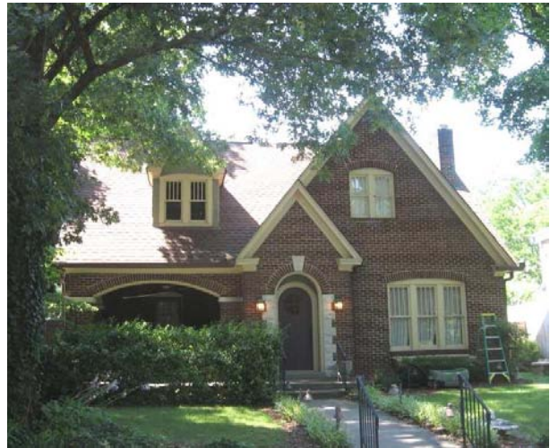
The grouped windows and quoin-like entrance surround at 810 West Main Street, as well as variously projecting bays, are typical Tudor Revival features.
