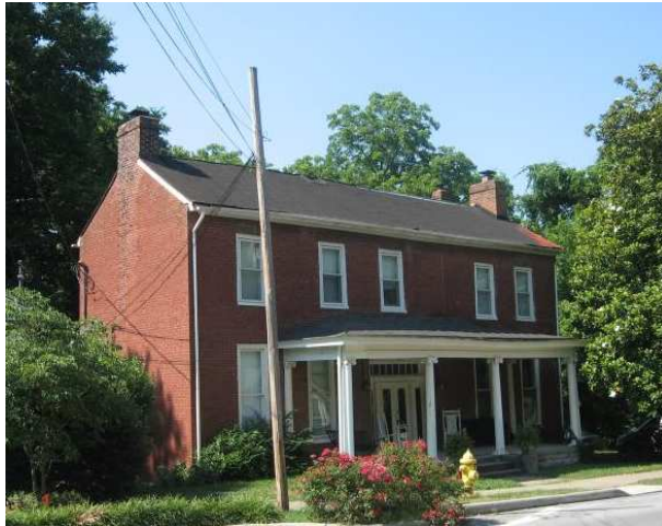
The chimneys at 724 Fair Street contribute to the balance so important to the house's Federal style.
