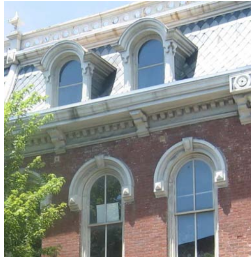
Window elements like the metal hoods at 346-348 Main Street contribute to historic character.
