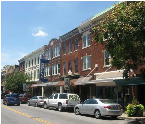
Flat roofs are a hallmark of historic commercial buildings.
