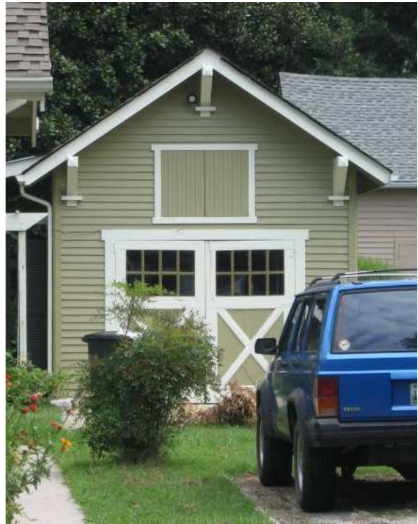
The small size relative to the house, traditional detailing and materials, and placement behind and to the side of the house make this garage at 217 Fourth Avenue South an appropriate model for infill garages.
