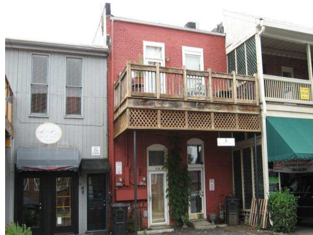
This deck at 420 Main Street used a simple design.
