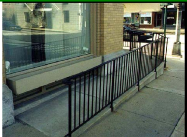
If access is needed for corner commercial buildings, consider using a side ramp and railing.
