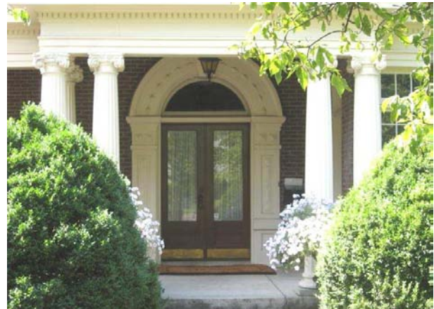
The original elaborate arched entrance and glass-and-wood doors at 812 West Main Street contribute to the house's historic character and should not be altered.
