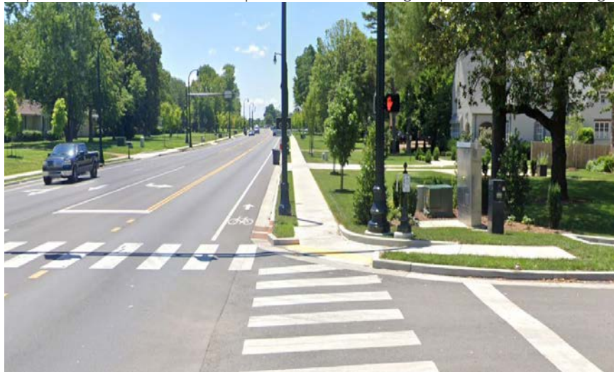
Existing bicycle lane on Hillsboro Road.
