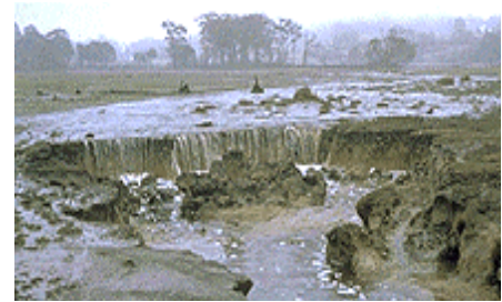
Severe Gully Erosion
