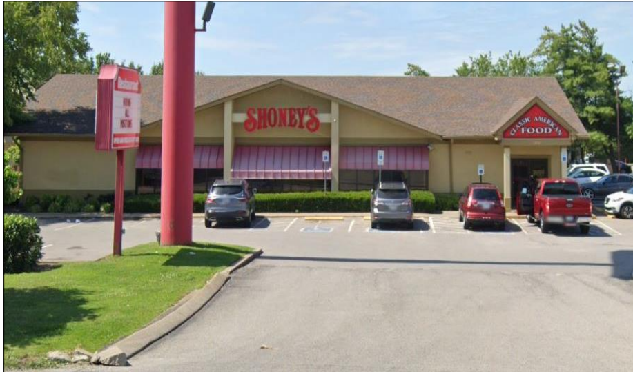
Current Building Located at 1306 Murfreesboro Road
