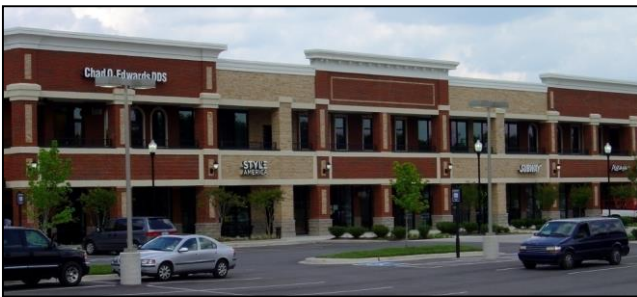
Figure 5-43: This building on a lot within a conventional area successfully uses arcades, wall offsets, and variations in roof line to break up the mass of the building and maintain a pedestrian orientation.
