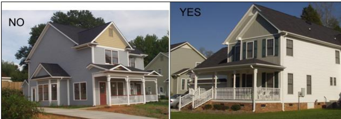
Figure 5-14: Residential structures incorporate raised foundations, as depicted in the photo to the right, to give a vertical orientation and well-proportioned appearance, as well as to provide privacy for occupants.
