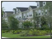
Figure 5-91: The image depicts how ground-based equipment located above grade can be screened from view.
