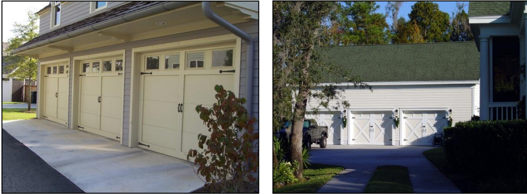
Figure 5-20: Street-facing garages that include a variety of architectural features help the garage blend with the dwelling and reduce garage-dominated views from the street.
