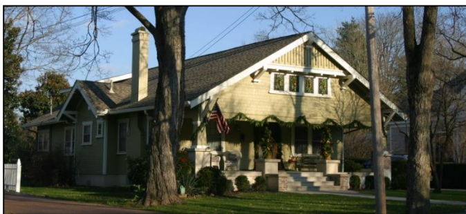
Figure 3-7: Example of a gabled roof with overhanging eaves as required in CAO 2.
