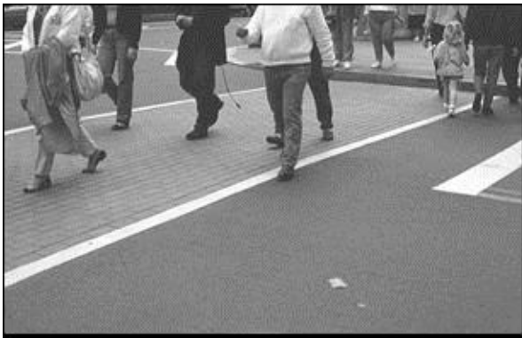
Figure 5-133: Textured pavers are an appropriate design element that can be used to accentuate pedestrian crossings.
