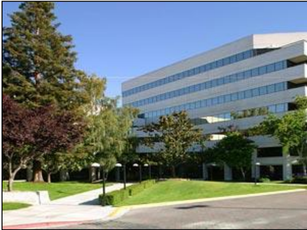
Figure 5-39: This image depicts a building with an orientation that is primarily horizontal, which is inappropriate for Franklin.
