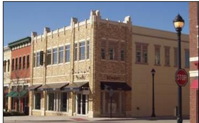
Figure 5-44: Flat roofs behind parapet walls with cornice treatments are appropriate for use within traditional areas.
