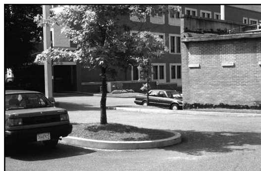
Figure 5-82: Curbing or other devices can help to define landscape islands in parking lots and help to limit damage to landscape materials by vehicles.
