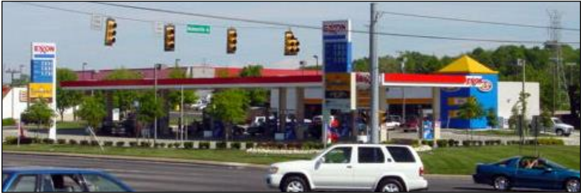
Figure 5-37: Corner lots on major intersections are inappropriate places for automobile fuel sales or similar automobile service and sales uses.
