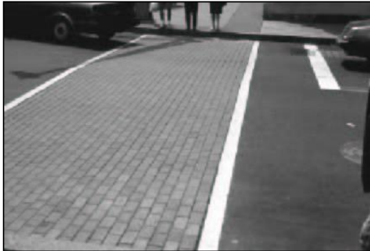
Figure 3-6: Example of a cross walk constructed of stenciled concrete. Pedestrian cross walks constructed of stenciled concrete, or an approved equivalent, enhance historic character CAO 2 and serve as a traffic-calming measure.
