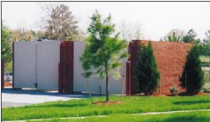
Figure 5-111: This image demonstrates how dumpster enclosures can be constructed of high quality materials and provide a completely opaque screen to a height above the dumpsters or recycling containers.
