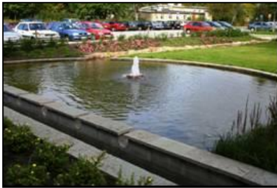
Figure 5-98: This image demonstrates how stormwater management devices can be integrated into a development site as an amenity feature.
