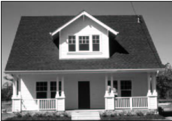
Figure 3-8: This house demonstrates vertically oriented windows, a raised foundation, and a front porch consistent with existing historic homes in CAO 2.
