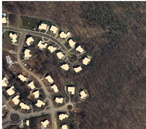
Figure 5-130: Cul-de-sacs are most appropriately used in areas of steep topography and where stream crossings are prohibited, as shown in this image.
