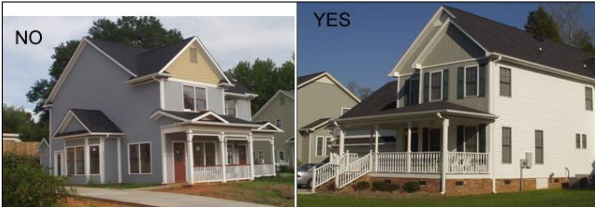
Figure 5-14: Residential structures incorporate raised foundations, as depicted in the photo to the right, to give a vertical orientation and well-proportioned appearance, as well as to provide privacy for occupants.
