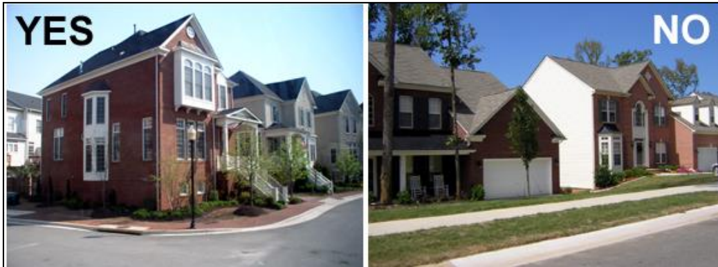
Figure 5-12: The Dwelling on the left demonstrates appropriate exterior wrapping, while the image on the right depicts a dwelling with inappropriate material changes at the corner of the building.
