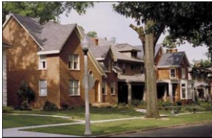
Figure 5-10: The detached dwelling in the foreground exhibits compatibility with the surrounding dwellings in regard to design, scale, setbacks, and materials.
