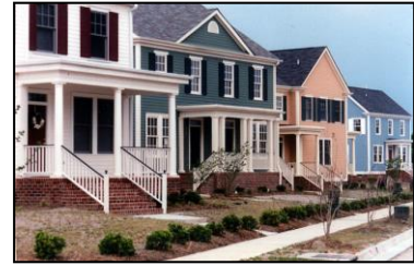
Figure 5-16: These homes demonstrate how heavier materials (brick) should be located below lighter materials (wood siding).
