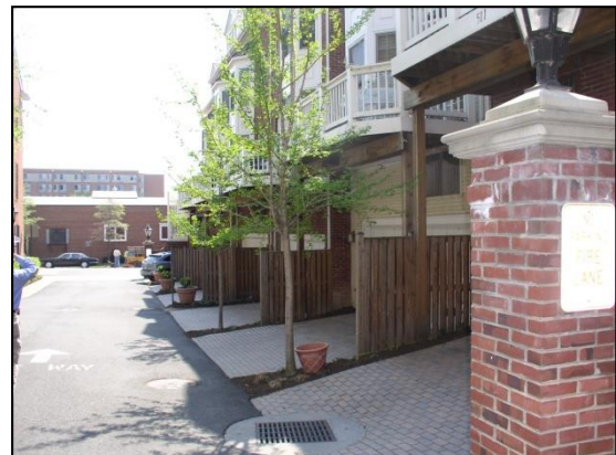
Figure 5-131: Alleys allow service functions to occur at the rear of dwellings and reduce the impact of cars, driveways, and garage doors on streets.
