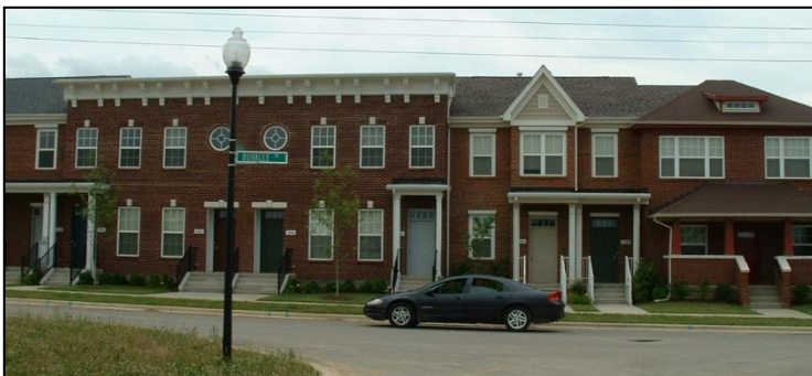
Figure 5-31: Roof forms can be used to denote building features such as entrances. Parapet walls can add visual interest through the use of a three-dimensional cornice treatment.
