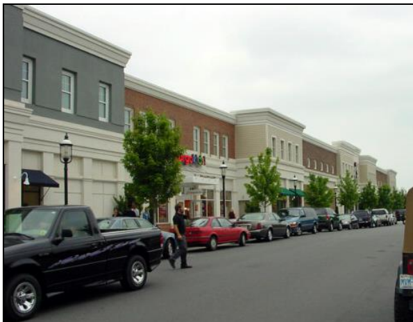
Figure 5-38: This building successfully blends the vertical height of the building with the horizontal banding of the base, middle, and cap.
