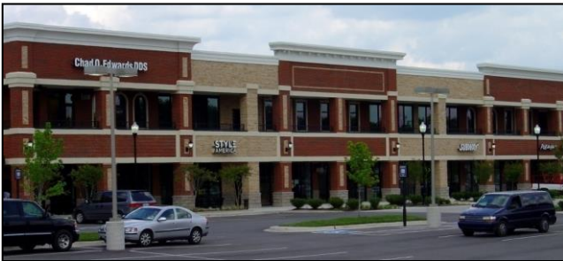
Figure 5-43: This building on a lot within a conventional area successfully uses arcades, wall offsets, and variations in roof line to break up the mass of the building and maintain a pedestrian orientation.
