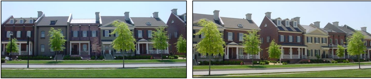
Figure 5-29: These attached residential structures demonstrate how different materials, changes in wall planes, offsets, projections, recesses, and other architectural techniques can promote variety in building façades.
