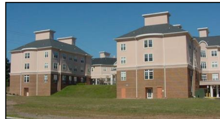
Figure 5-28: This attached residential development lacks sufficient façade variation yielding a monotonous appearance.
