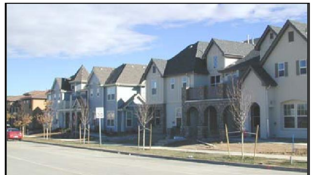
Figure 5-27: This image demonstrates how an attached residential structure of six or fewer units can be constructed to appear as a large detached residential structure.
