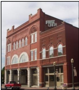
Figure 5-42: This building uses pilasters to divide a single façade into distinct vertically-oriented storefronts that maintain the building rhythm along the street.
