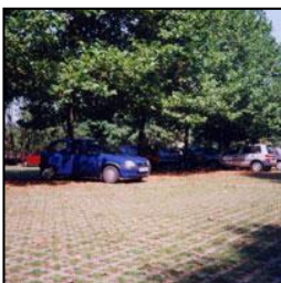
Figure 5-124: Pervious or semi-pervious surfacing materials such as grasscrete or grasspave may be used as an alternative surfacing material for surface parking areas.
