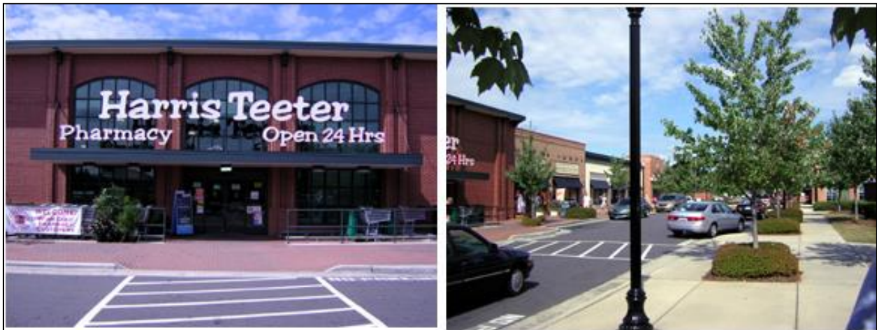
Figure 5-122: Primary drive aisles are designed to appear as an extension of the public street network through the inclusion of sidewalks, “street” trees, and parallel parking spaces where appropriate.
