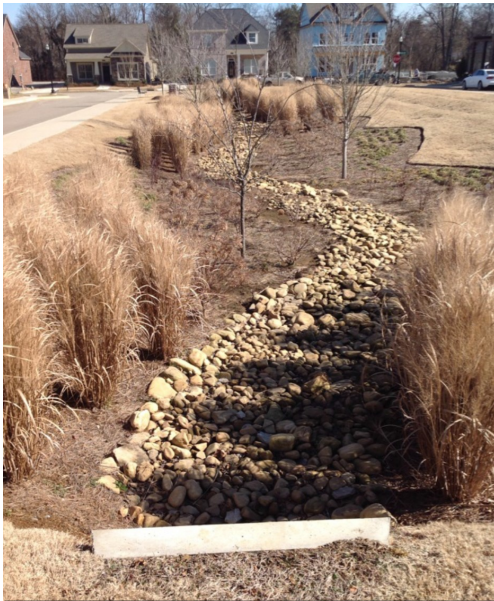
Bioretention cell at Tywater Crossing Subdivision
