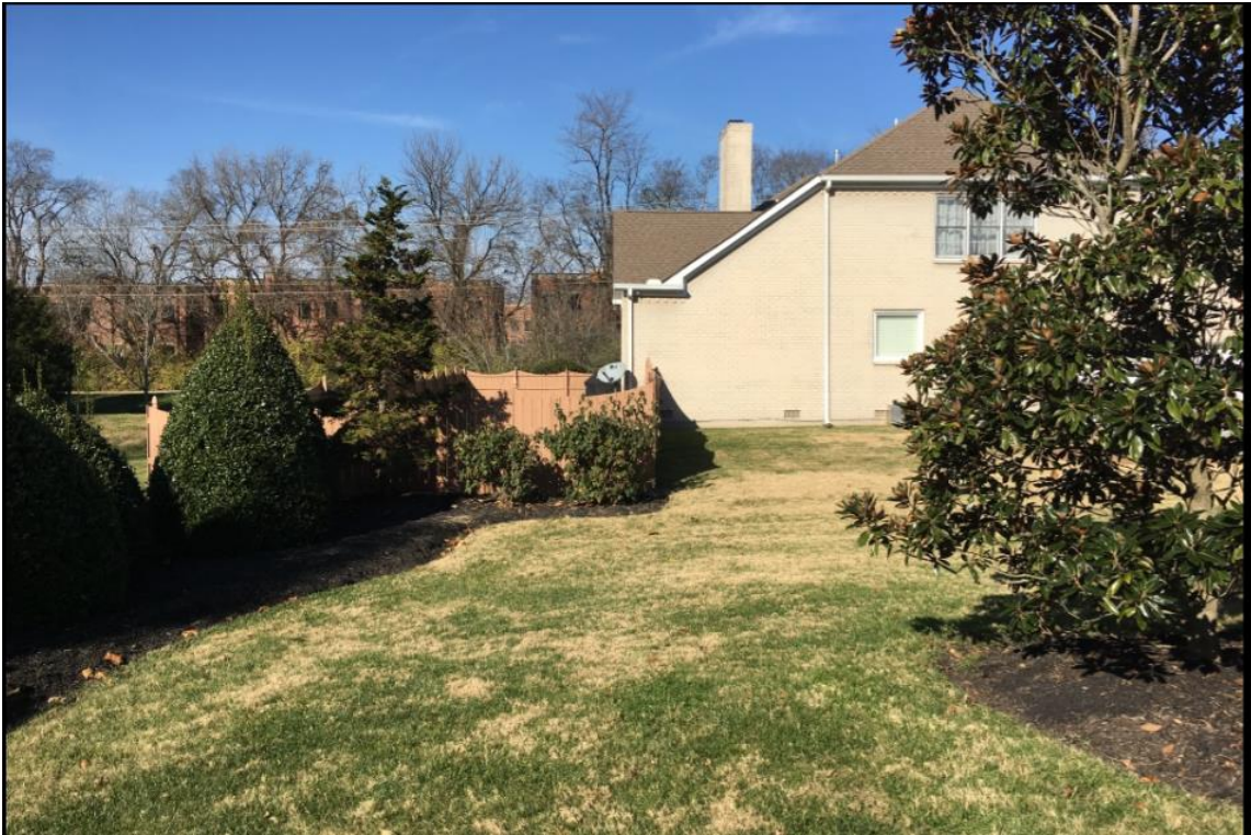
Picture 5. North view from the existing slab, future covered screen porch.
