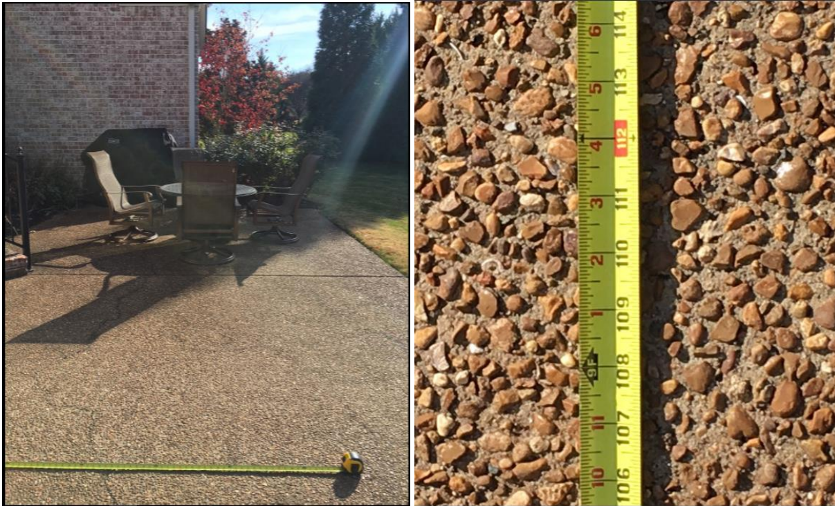
Picture 3. End of 40' Rear setback at end of wall, only 9' depth.
