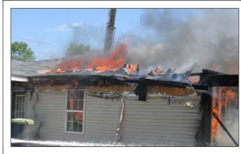
West Main St. house fire.
