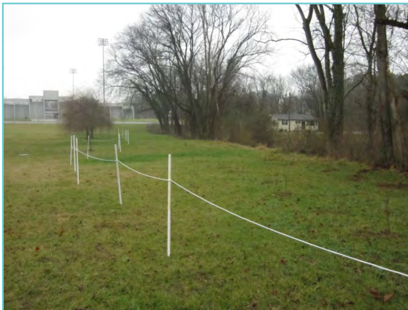
Figure 33. Temporary fencing to protect newly installed seedlings at South Doyle Middle School on Baker Creek, Knoxville, TN
