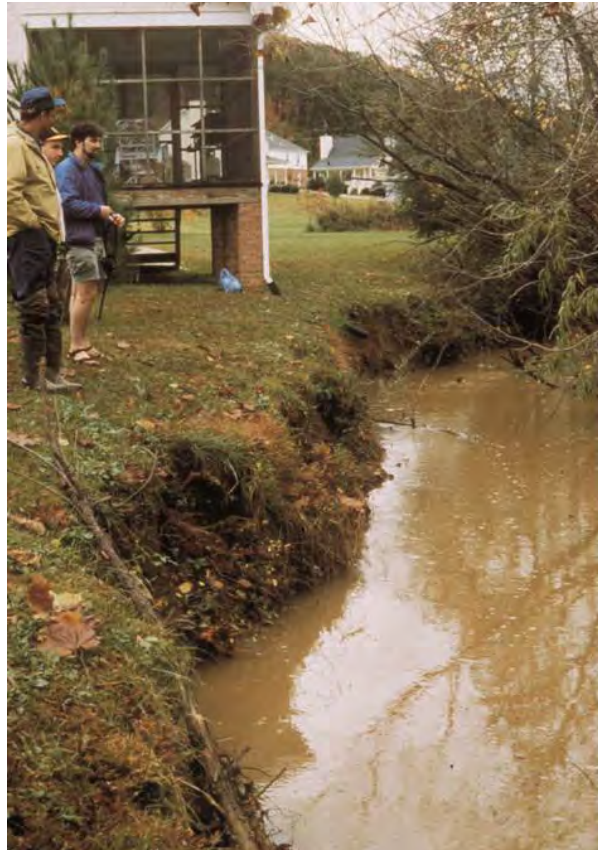
Figure 7. Severe streambank erosion in urban setting
