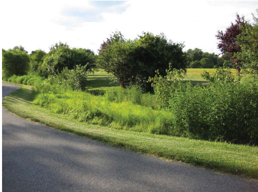
Figure 5.1. Water Quality Swale w/ tall meadow grasses & herbaceous plants along trail receiving runoff from parking area (source: National Transportation Enhancements Clearinghouse / www.enhancements.org )
