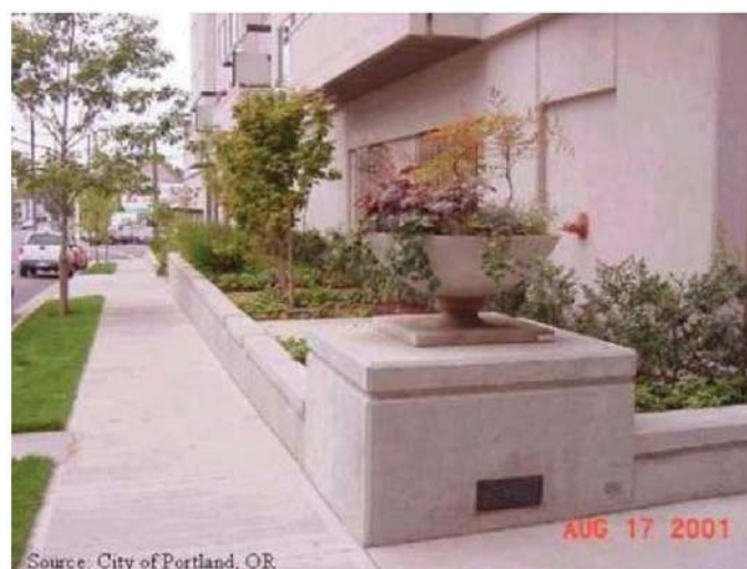
Figure 2.1. Stormwater Planters (source: City of Portland, OR)
