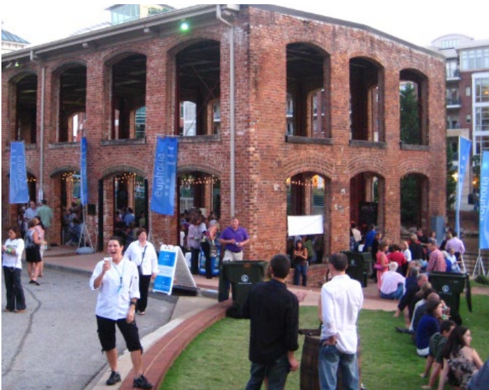
Example of floodable structure
