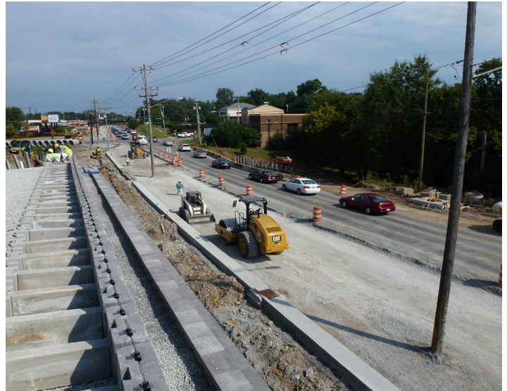
Hillsboro Street Improvement Project
