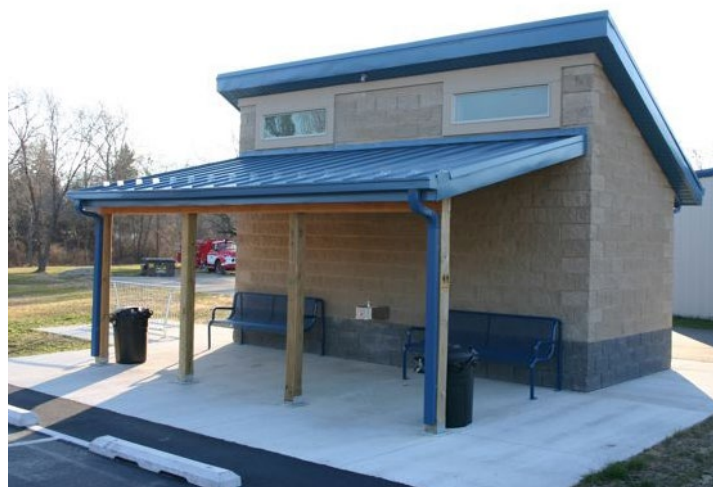
Example of open pavilion
