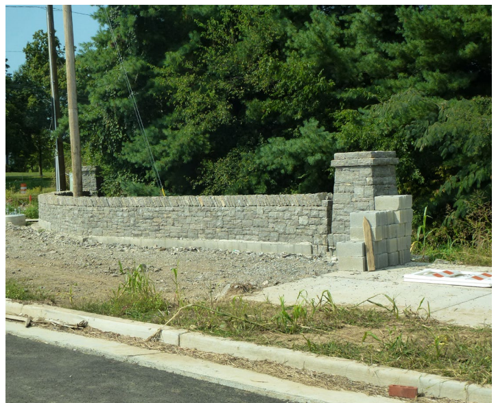
New 3rd Avenue culvert bridge
