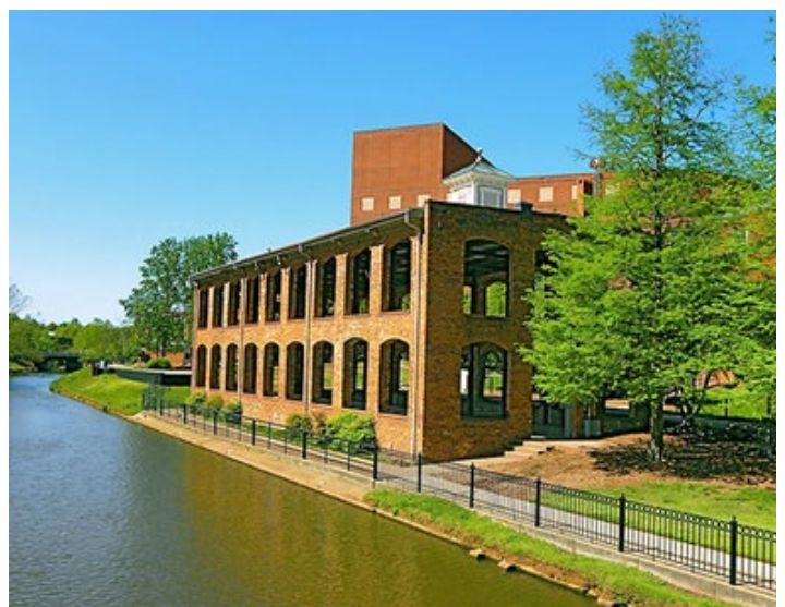
Example of floodable structure
