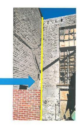
Option 2: Remove damaged wall above counter flashing and cap with metal to create a small parapet wall and paint to match existing roof vents.
