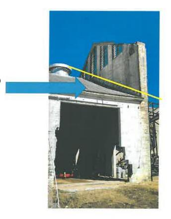
Option 2: Remove damaged wall below the vented gable to create a flat top parapet and will have a metal flashing placed on top and paint to match existing roof vents. This could act as a point if a discussion was needed or fact that the space beyond this onced boused the boiler
