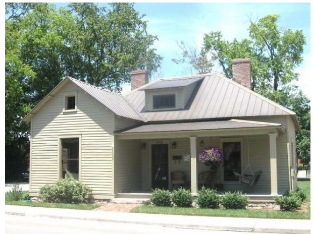
Should wooden siding like that at 202 Church Street require replacement, the historic materials should be used as a model.
