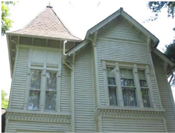
The decorative siding on the house at 819 West Main Street contributes to its Queen Anne character.
