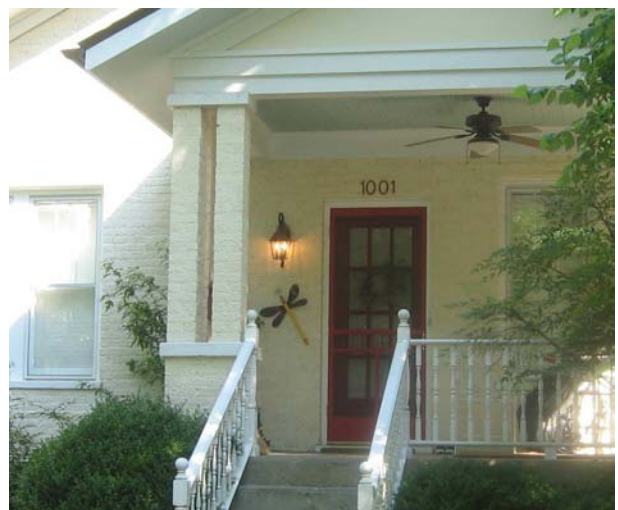
Both the wall and ceiling fixtures at 1001 Fair Street are appropriately placed.
