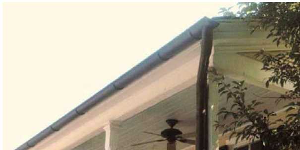
The gutter at 117 Seventh Avenue North uses an appropriate half-round design.
