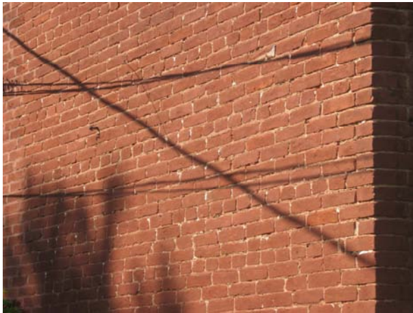
Brick is one of Franklin's primary historic building exteriors (724 Fair Street).
