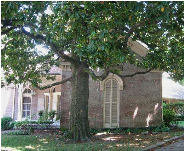
The arched, crowned openings on 805 West Main Street are typical Italianate features.
