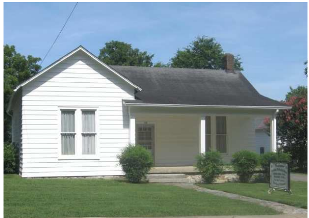
Property owners are encouraged to remove synthetic siding and restore the original wood siding (1326 Adams Street).
