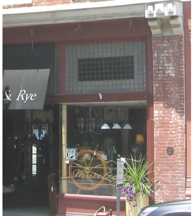
The building at 346-348 Main Street retains original storefront elements, including decorative transom glass.
