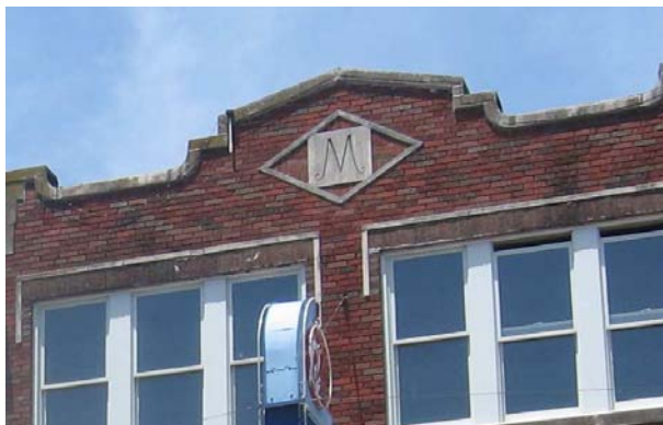
Parapets, coping, and ornaments, like those on 332 Main Street, contribute to historic character.
