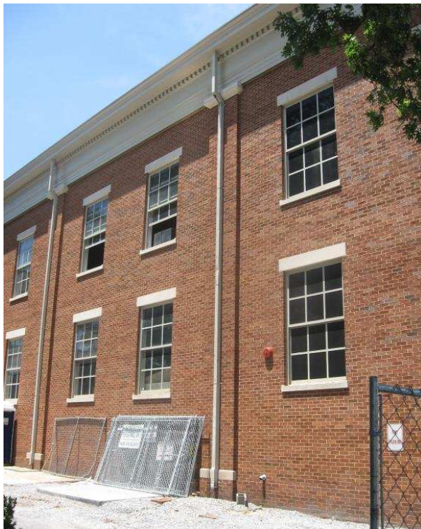
Gutters and downspouts, like these on the courthouse, help protect buildings from water damage.
