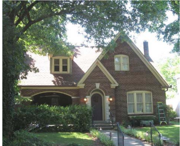
The grouped windows and quoin-like entrance surround at 810 West Main Street, as well as variously projecting bays, are typical Tudor Revival features.
