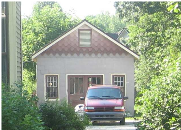
Details like original doors and windows contribute to the character of this outbuilding at 1004 Fair Street.
