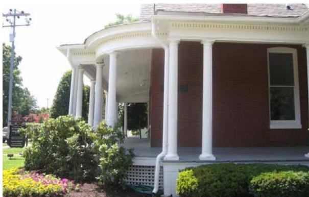
The downspout on 143 Fourth Avenue North uses placement at a corner and coloring that matches its adjoining surface to minimize its visual effect.
