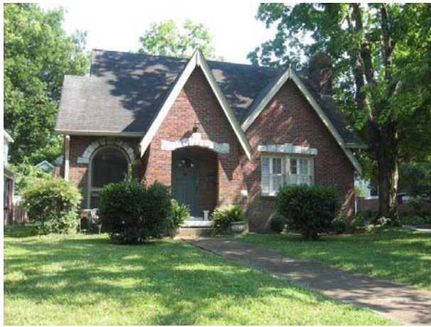
The house at 809 Fair Street includes many Tudor Revival features; the multiple steep gables and varied surface treatments are prime examples.
