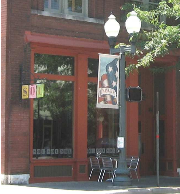
Large display windows and bulkheads beneath them, like these at 401-403 Main Street, are traditional storefront elements.
