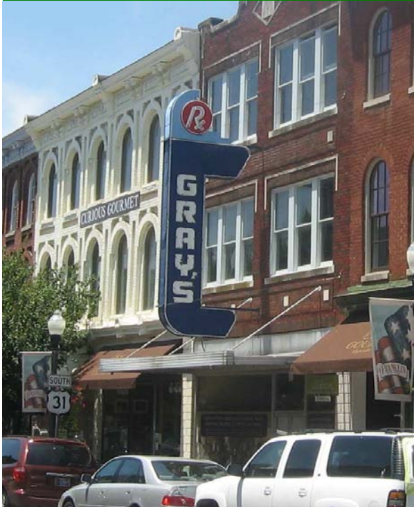
Historic signs like this one at 332 Main Street contribute to district character.
