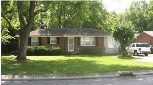
This house at 1251 Adams Street has the horizontal emphasis, rectangular form, and simple exterior of the Ranch style.
