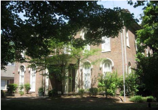
Unpainted masonry was common for Italianate buildings like this one at 123 Fifth Avenue North.
