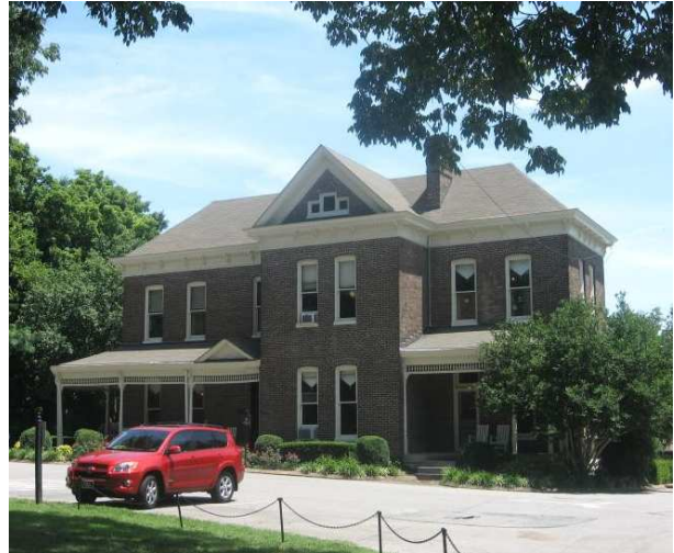
The house at 150 Franklin Road, now part of Battle Ground Academy, is a restrained example of the Queen Anne style. It has varied surface planes, one-over-one windows, and full-width porches with milled trim and posts.
