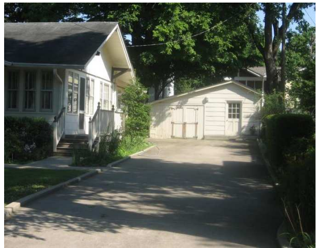
The placement of this garage at 1009 Fair Street, alongside and recessed from the house, is typical.
