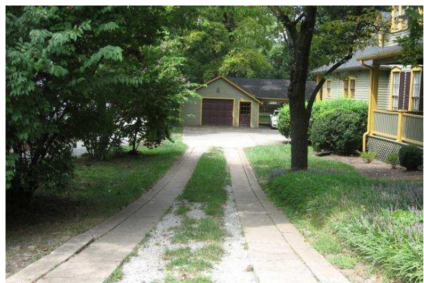
Split driveways like this one at 108 Lewisburg Avenue are common historical designs and are also helpful in addressing the problems of runoff.
