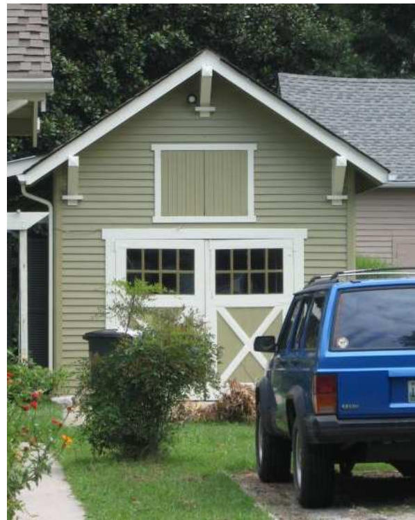
The small size relative to the house, traditional detailing and materials, and placement behind and to the side of the house make this garage at 217 Fourth Avenue South an appropriate model for infill garages.
