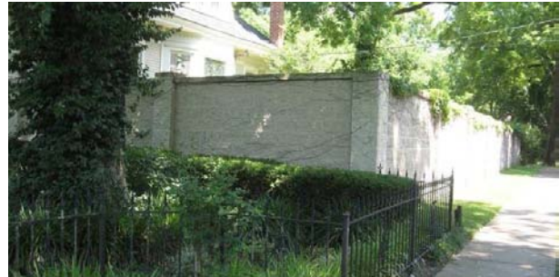
Solid walls like this one at 1059 West Main Street are only acceptable for rear and side yards.
