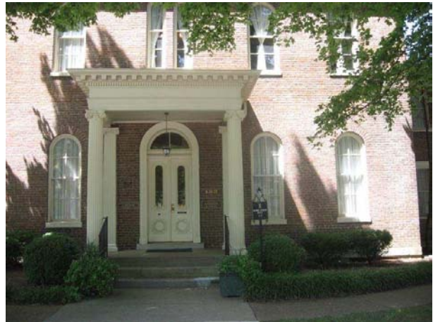
The small porch on a side elevation, paired wooden doors with large single panes, and arched openings on 123 Fifth Avenue North are all Italianate features.
