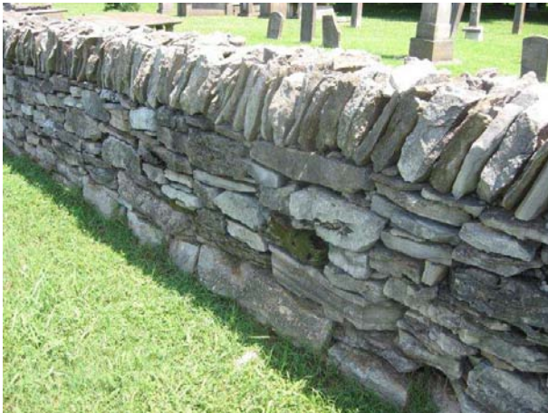
Historic stone walls like this one on Fourth Avenue North around the City Cemetery should be preserved.
