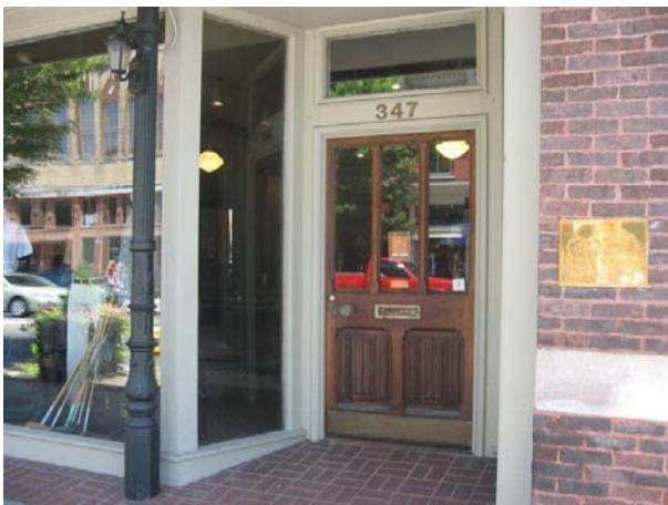
At 347 Main Street are original columns and recessed entrance.
