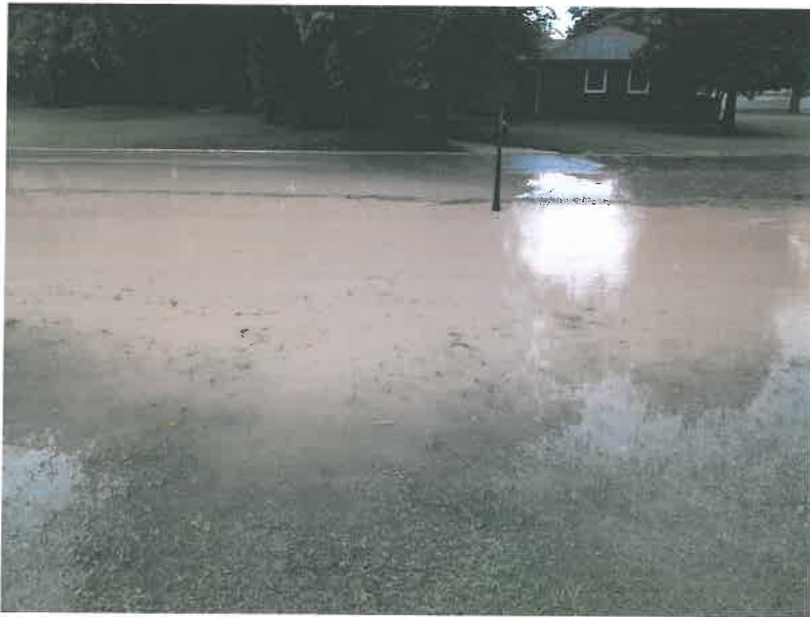
403 Figuers Drive – Flooding on 08/11/13
