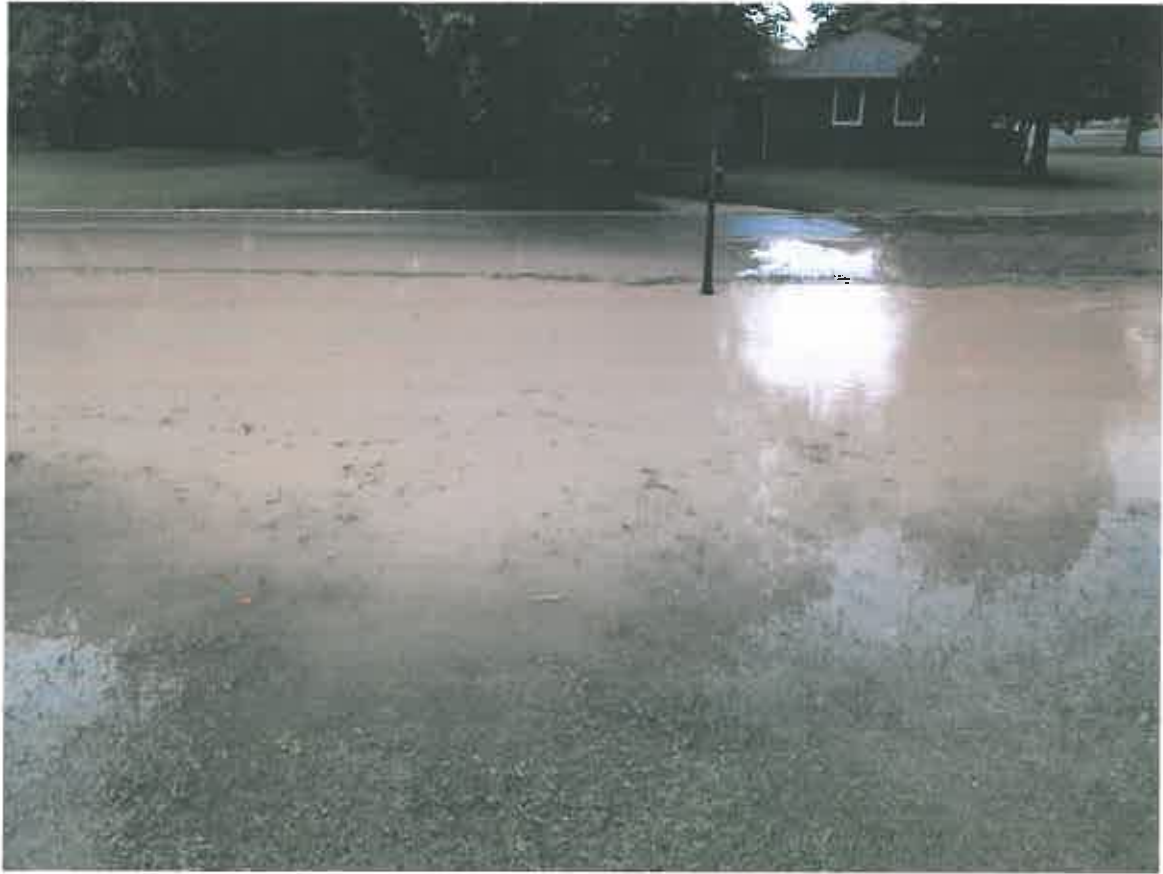
403 Figuers Drive – Flooding on 08/11/13
