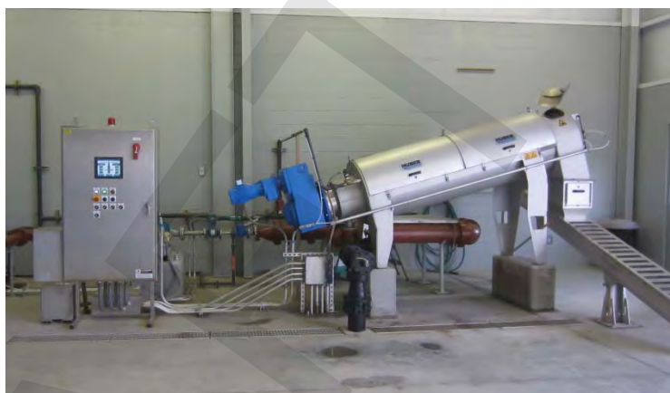
Figure 3 Huber Technology Screw Press Installation in Blairsville, GA
