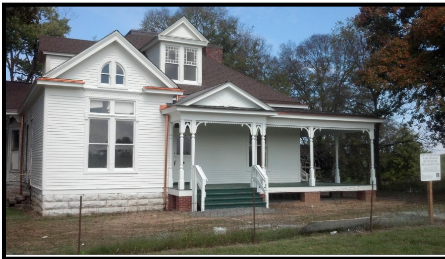
2012: Pre-Construction Picture of the Historic Hayes Home
