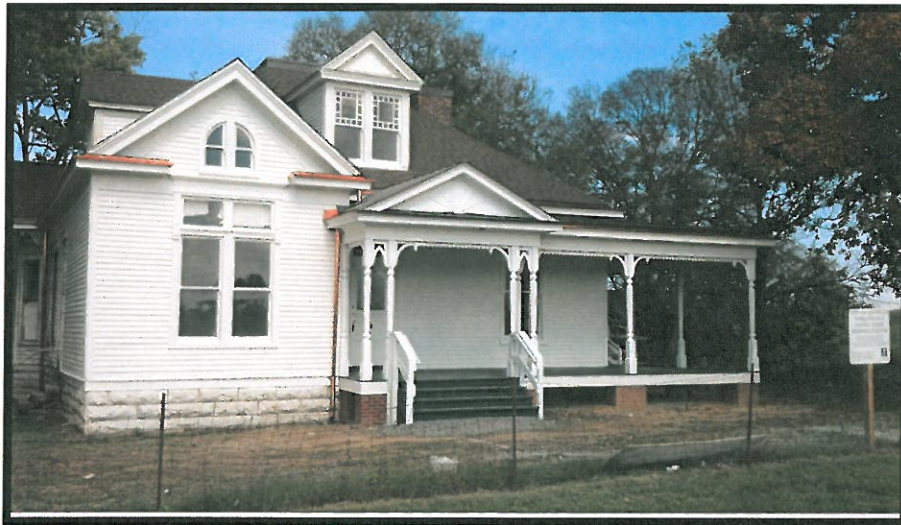
Post Completion of Weatherization & Restoration of the Historic Hayes Home Project 2012.
