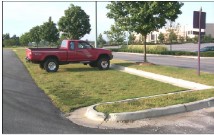
Grass Paver Surface Used for Parking
