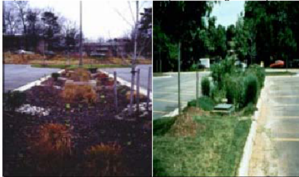
Profile of Parking Lot Bioretention Facilities
