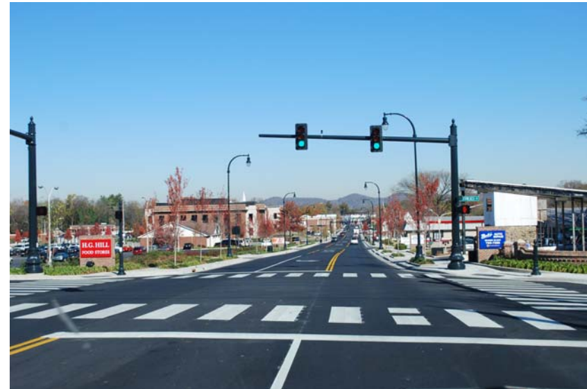
Columbia Avenue AFTER Streetscape.
