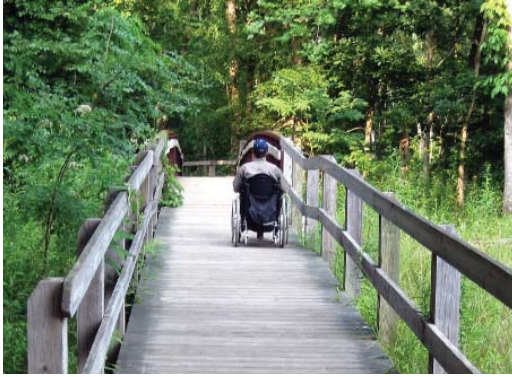
Accessible bridge crossing at wetlands
