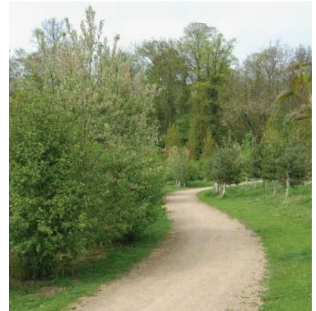
Trail designed with pervious pavement
