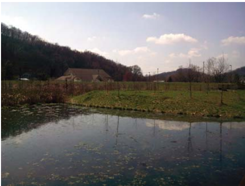
Constructed wetlands on the corner of Franklin Rd. and Moores Ln.
