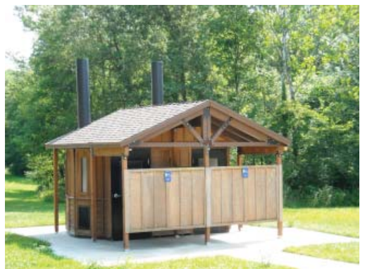
Example of a restroom facility
