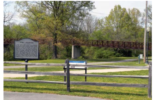
Pedestrian bridge at Pinkerton Park
