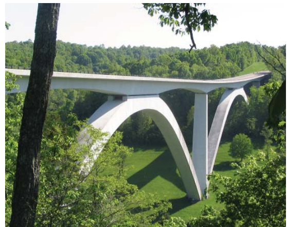
The Natchez Trace Parkway Bridge
