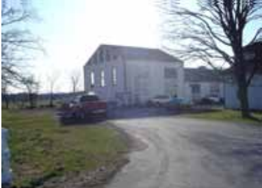
Former power station plant
