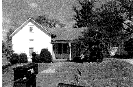
236 Third Avenue N Office Residential, FFO
