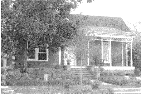
245 Third Avenue N Office Residential, FFO
