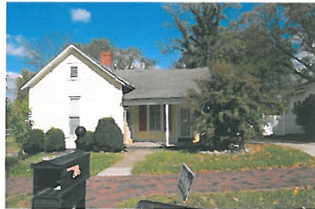
236 Third Avenue N Office Residential, FFO
