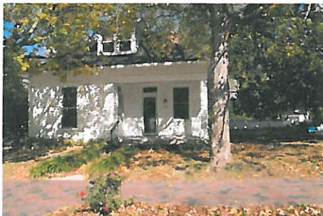
232 Third Avenue N Office Residential, FFO
