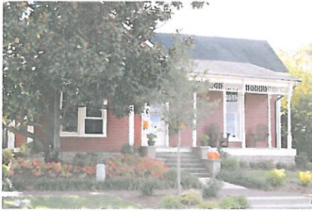
245 Third Avenue N Office Residential, FFO
