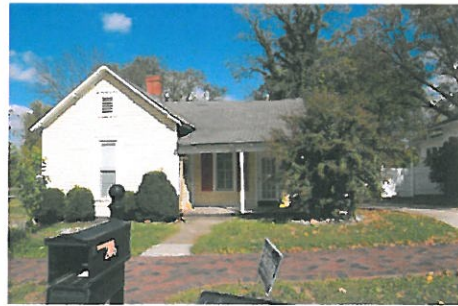
236 Third Avenue N Office Residential, FFO
