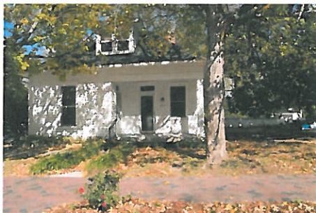
232 Third Avenue N Office Residential, FFO
