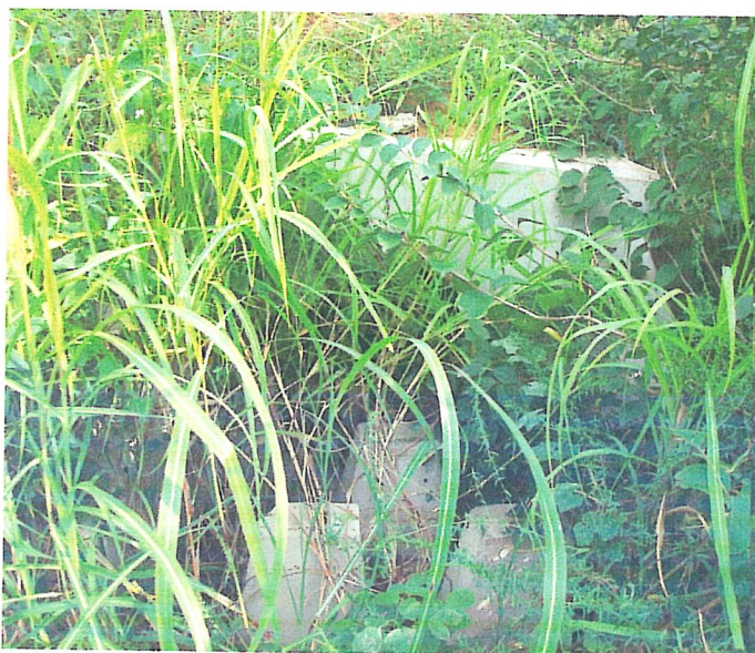
Energy dissipater Headwall outfall facing north
