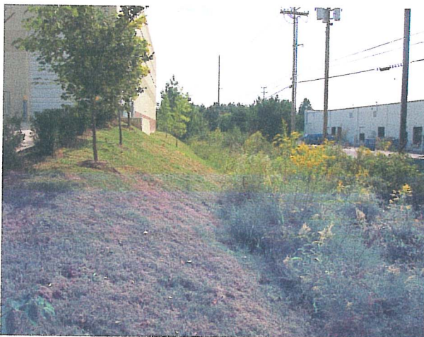
Swale: Facing east (from back of building to front)
