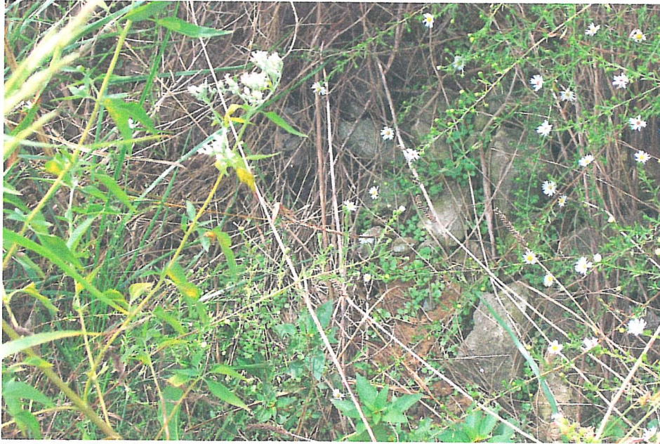
Bottom of swale near energy dissipating headwall
