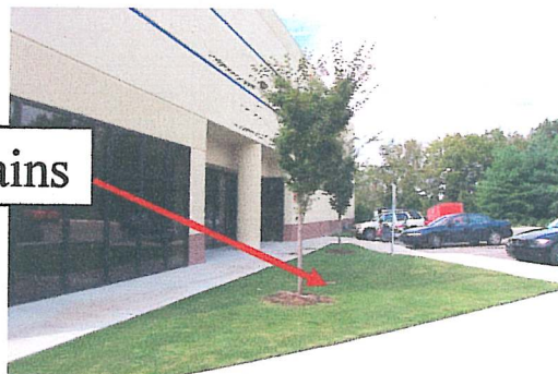
Storm drain on north side of building. It drains the small green area.
