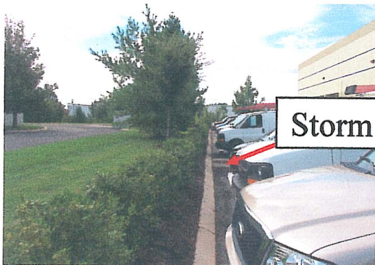
Storm drain on east side in car parking lot. It drains the entire parking lot.
